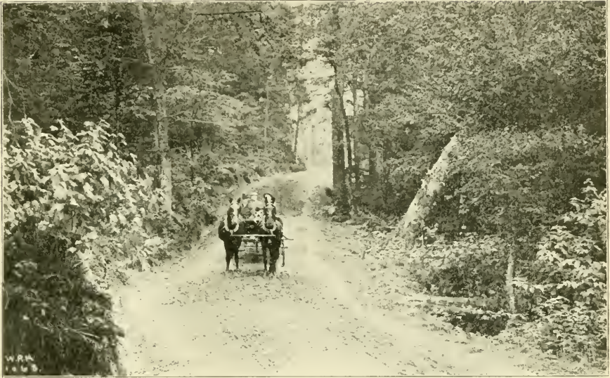
A Section of the Jefferson Notch Road.
