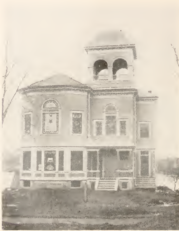
Public Library Building.
