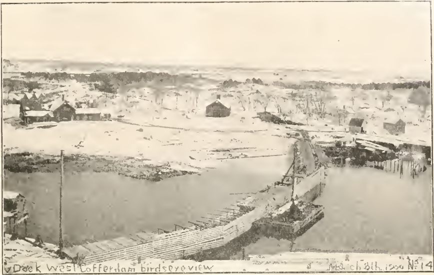
Coffer-dam under construction at the mouth of the proposed new dry dock, and which recently broke away beyond the far-off angle to be seen in the illustration. Photographed March 8, 1900.
