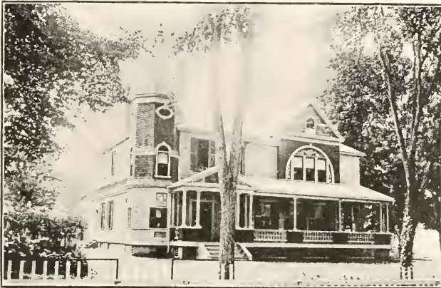
Hastings Memorial Parish House.
