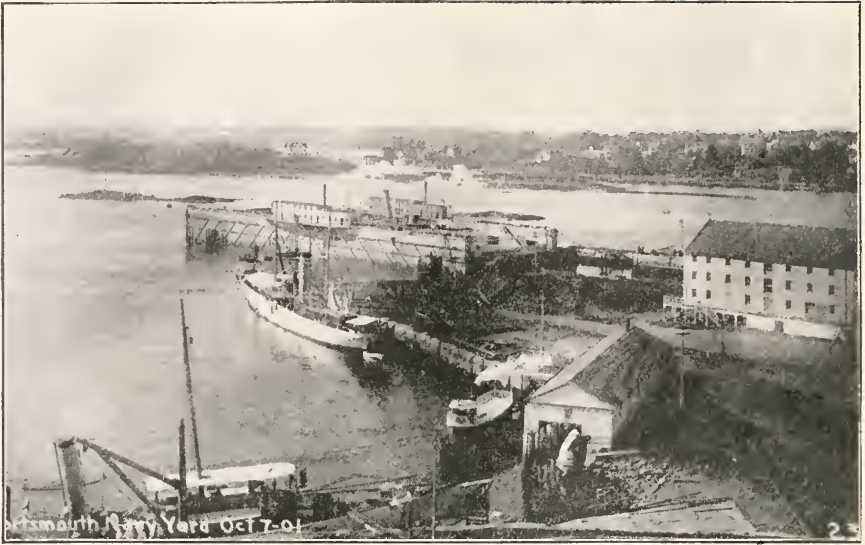
View showing wooden dry dock, built in 1852, having a vessel docked (U. S. S. Iiven ), Kittery and Badger's island in the distance, October 7, 1901.
