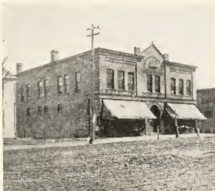
The Rollins Building.
