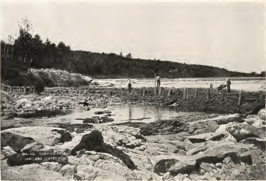
This shows one of several sand-bag coffer-dams which turned the river from side to side, as desired.
