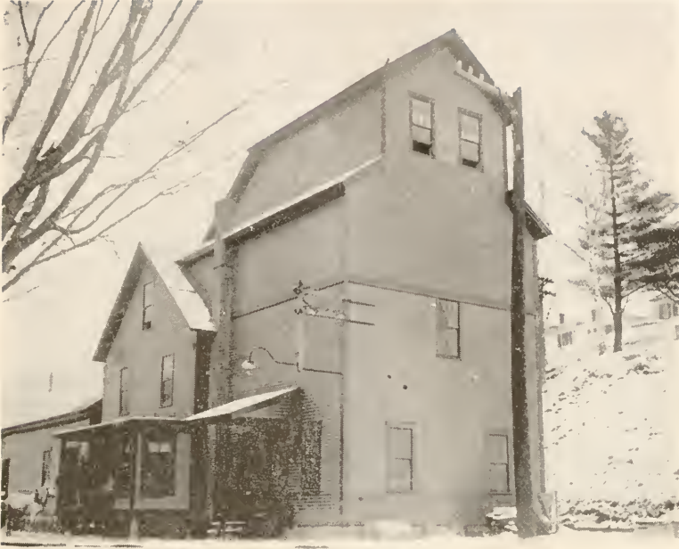
Grain Elevator of Wells &amp; Flanders.
