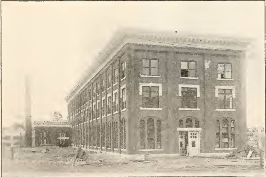
New $100,000 equipment building at the head of the dock, having Concord granite for trimmings. June 29, 1903.
