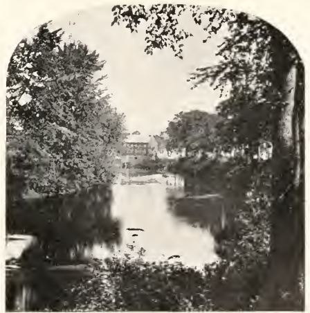
River View, with Old Mill and Dam.
