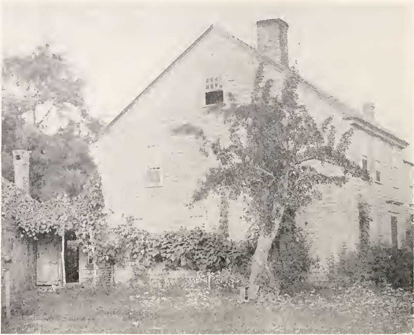
Locust Grove House, looking towards Spring Hill.
