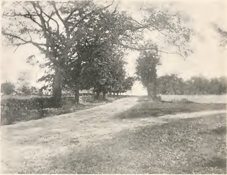
Section of Highway leading from Nottingham to Epping.
