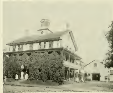
New Hampshire Central House.
