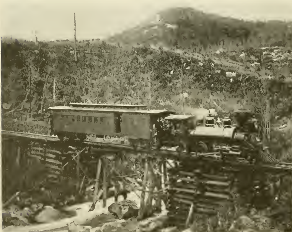
The Highest Trestle on the Zealand Valley Railroad.
