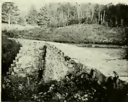
Wall of Reservoir.
