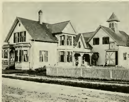
Residence of Frank Hadley.
