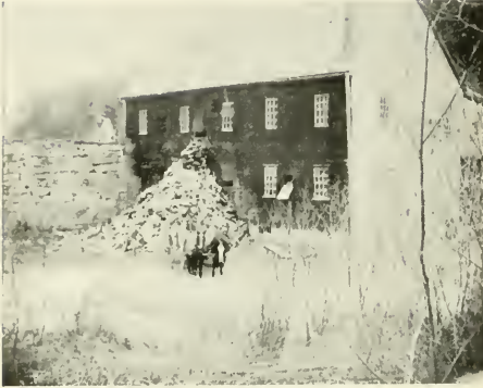
Site of Sawmill where Lumber was Sawed for the Church in 1804.
