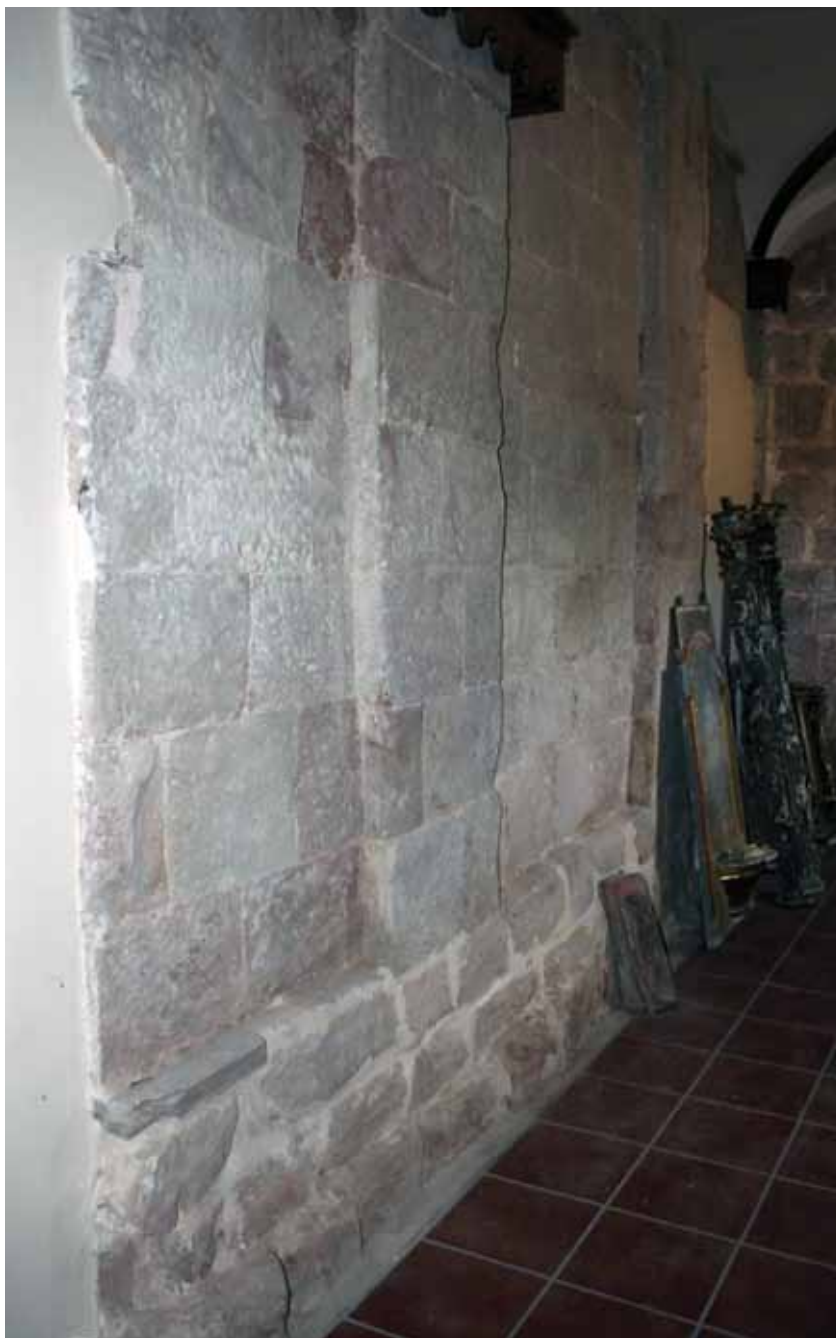
ILLUSTRATION 15. SANTA MARÍA DE VILLAVELAYO: BLIND ARCHES THAT RUN ALONG THE NORTH WALL (PHOTO: FÉLIX PALOMERO).
