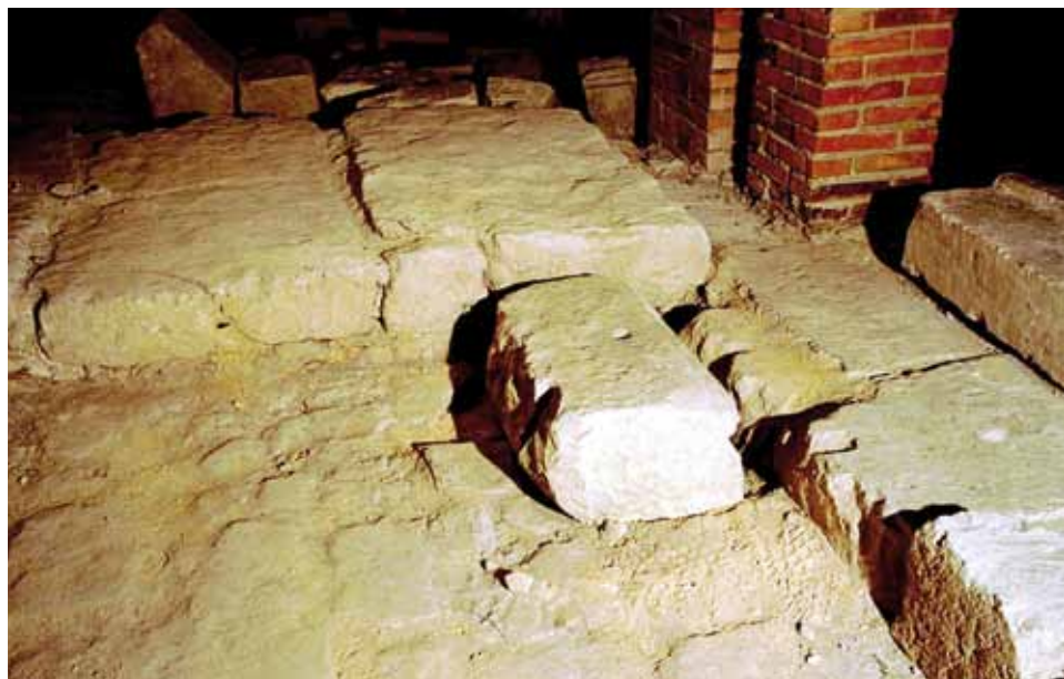
ILLUSTRATION 6. SANTO DOMINGO DE SILOS: NORTH WALL OF THE LOW CHURCH AND FOUNDATION OF THE TOWER (PHOTO: FÉLIX PALOMERO).
