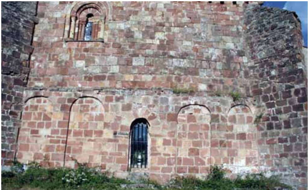
ILLUSTRATION 13. SANTA MARÍA DE VILLAVELAYO: BLIND ARCHES THAT RUN ALONG THE WEST WALL (PHOTO: FÉLIX PALOMERO).
