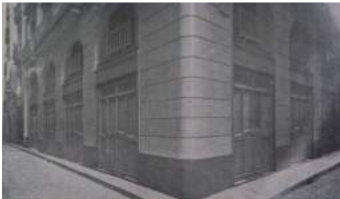
Dispensari 1 de Barcelona (c/ Rauric, 18)
