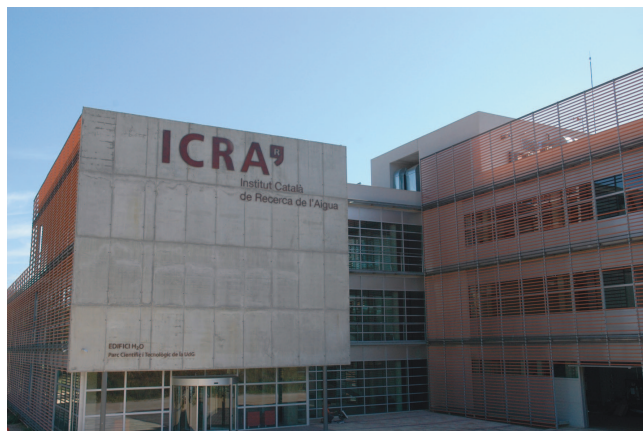
Fig. 1. External view of the ICRA's H2O building.
