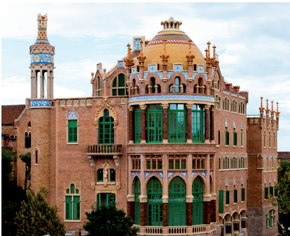
Fig. 1. Sant Manuel Pavilion of the Sant Pau Art Nouveau Site, designed by Lluís Domènech i Montaner and build under the direction of his son, Pere Domènech i Roure, in 1923. (Photo by Robert Ramos © Fundació Privada Hospital de la Santa Creu i Sant Pau).
