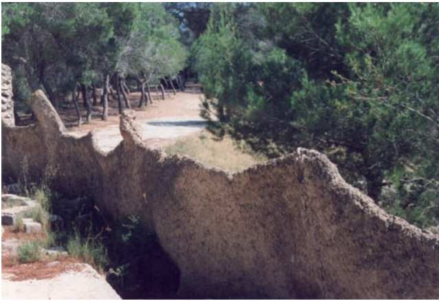
Fig. 14. Monserratina fence, built with a bedsprings frame by Josep M. Jujol in Montferri (1922).
