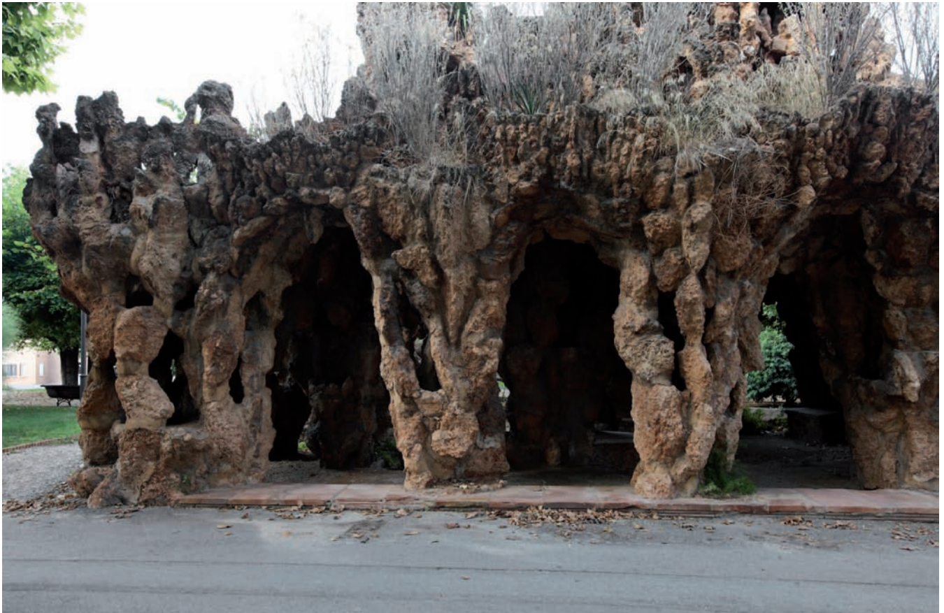
Fig. 7. Perimeter pillars of the Cova Cascada.
