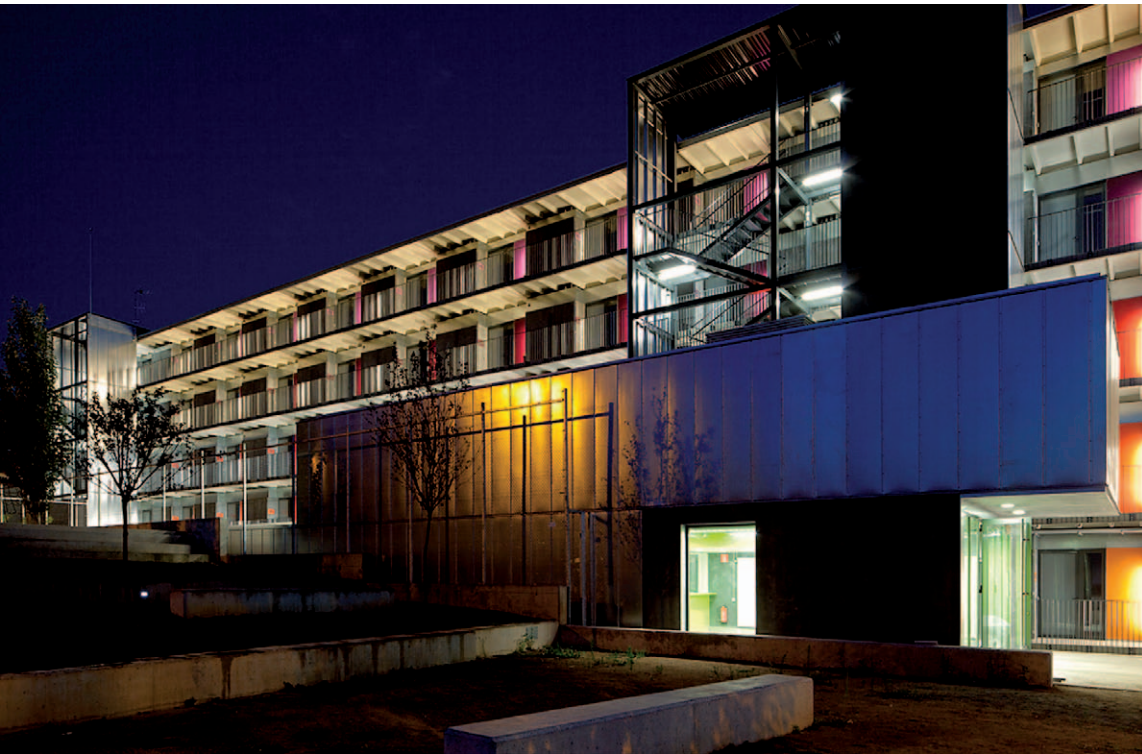
▲ University Housing at the Manresa Campus - FUB / EPSEM / UOC. Location: Manresa University Avenue #12. Manresa (Barcelona). Commissioned by: City of Manresa. Builder: Constructora d'Aro. Architect: Xavier Tragant. Number modules: 75 units. Total constructed area: 4,110 m 2 . Total module constructed surface: 56 m 2 . Module dimensions: 11.20 x 5.00 x 3.18 m
