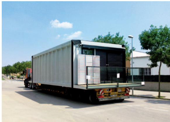
▲ Transport and assembly of industrial modules
