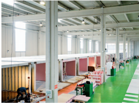
▲ Industrial module assembly line. Specialised and organised work areas along the assembly line are fixed and the modules move at a steady pace
