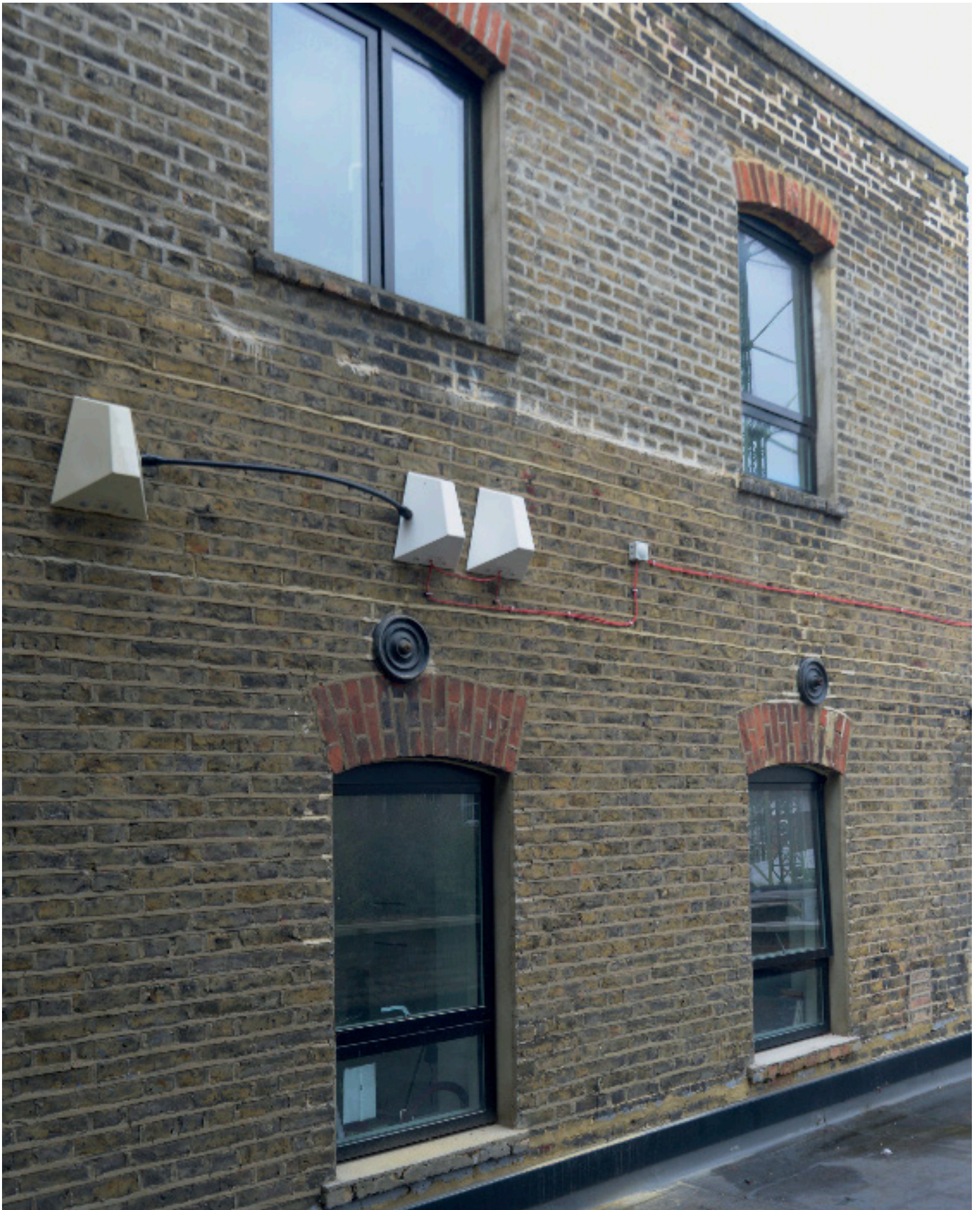
Figure 4. Interlocutor (2018). External installation of the Vacuum formed high-impact polystyrene, electrical components.
