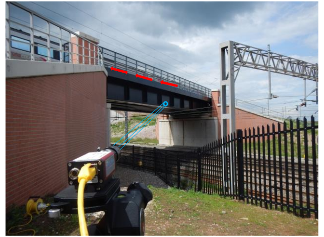
Figure 5. Videogrammetry system setup for measuring midspan deflection of east main girder
