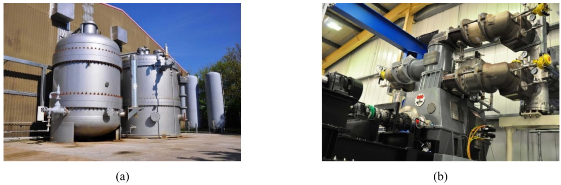
Figure 17. Views of the: (a) packed-bed thermal stores; and (b) reversible reciprocating compression/expansion machine of the PTES system demonstrator developed by Isentropic Ltd and completed by Newcastle University [109].
