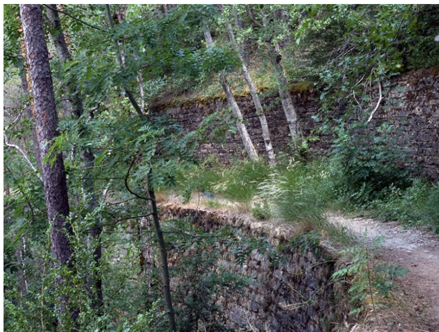
Figure 4. Stabilization terraces in the Arratiecho watershed.
