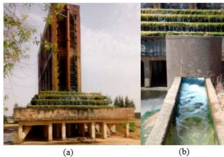
Figure 2. (a) Cooling system (b) irrigation canal.
