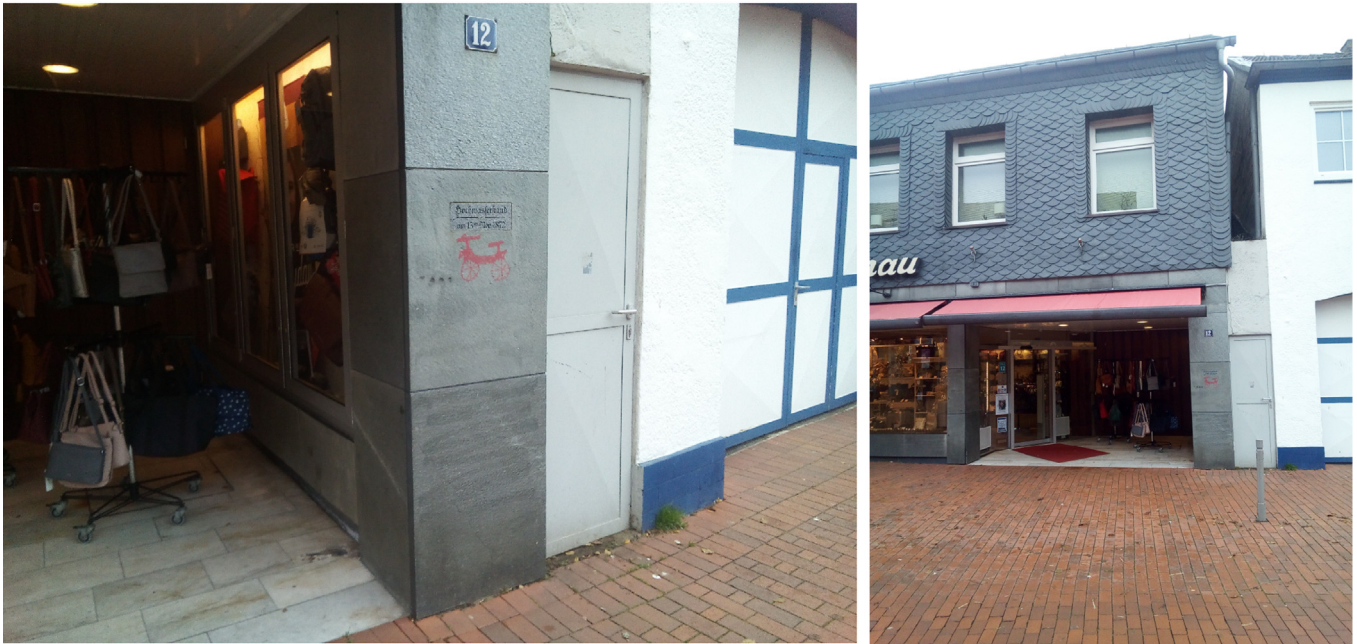
Fig. 2. Storm flood mark in Eckernförde, left picture with the mark of 1872, right with the entire house (Photographed by Michael Packschies, November 2019).
