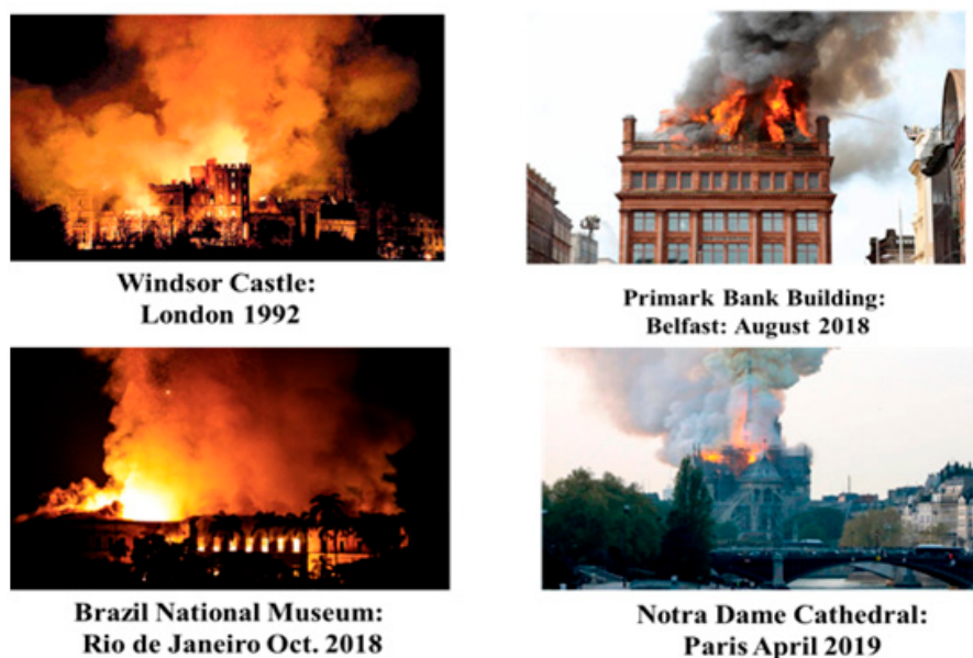
Figure 8. Catastrophic building fires that occurred after or during roof refurbishment where aluminum paneling may have played a role.
