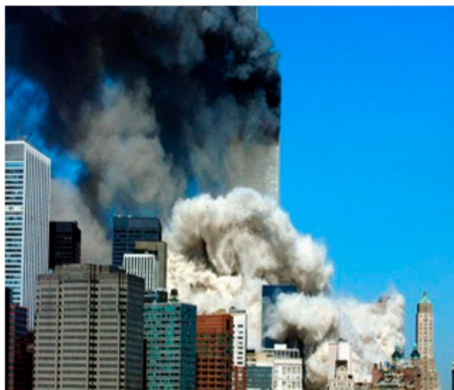
Figure 7. Collapse of New York World Trade Center 11 Sept. 2001.
