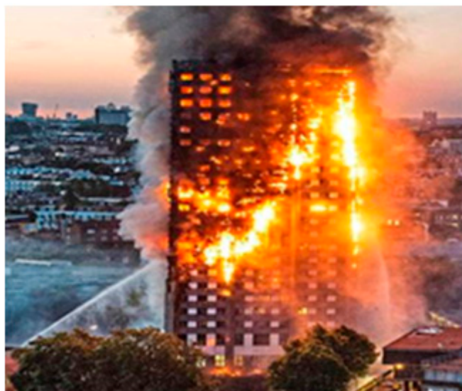
Figure 1. Burning Grenfell Tower at the height of conflagration; the black smoke at the top is combustible material burning without water; the whitish gas is mainly alumina dust from the reaction of Al and or Al_4C_3 and steam, as the water still being applied. Note the intensity of the conflagration where the water hits the building, and the associated whitish clouds around.
