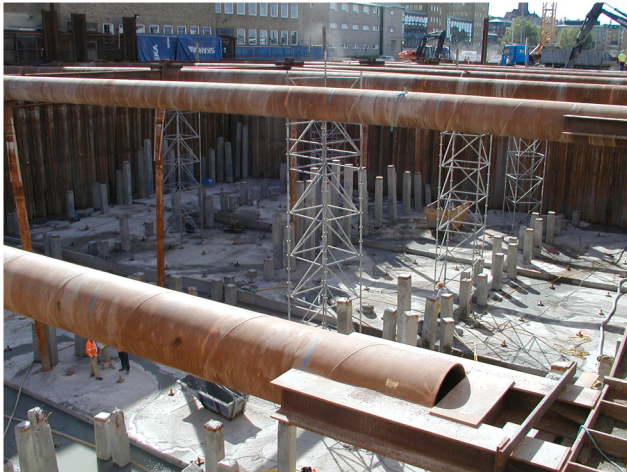
Fig. 5. The excavation after final dewatering in August 2003.
