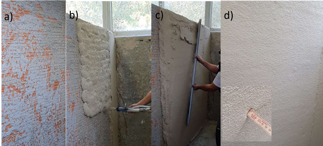
Figure 2. Photos showing the application steps of AP on a demo wall. a) Undercoat layer is smeared onto the surface. b) AP is sprayed on the surface until the desired thickness is achieved. c) The surface of the applied AP is smoothed. d) The final exterior appearance of the AP after the application.
