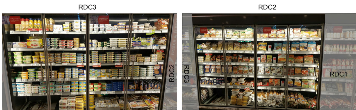
Fig. 1 Photos from the investigated supermarket, showing the neighbouring refrigerated display cabinets, RDC_2 and RDC_3
