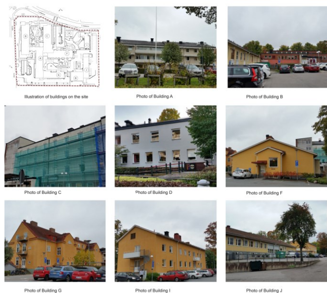
Figure 2. Photos of existing buildings
