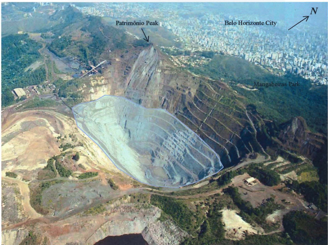
Plate 7 – Planned Final Configuration of the Pit's Lake. The easy access to the lake through Mangabeiras Park, the altitude and the steep slopes make the locale a potential risk for people. (Plate Courtesy MBR).
