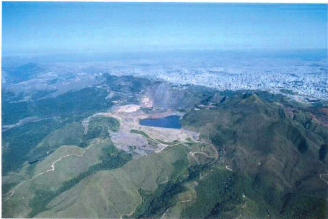
Plate 1 – Águas Claras Mine aerial view showing Belo Horizonte City, the pit, waste dumps Grota 2 and 3, the PFF dike and part of the Jambreiro Forest. (Plate Courtesy MBR)
