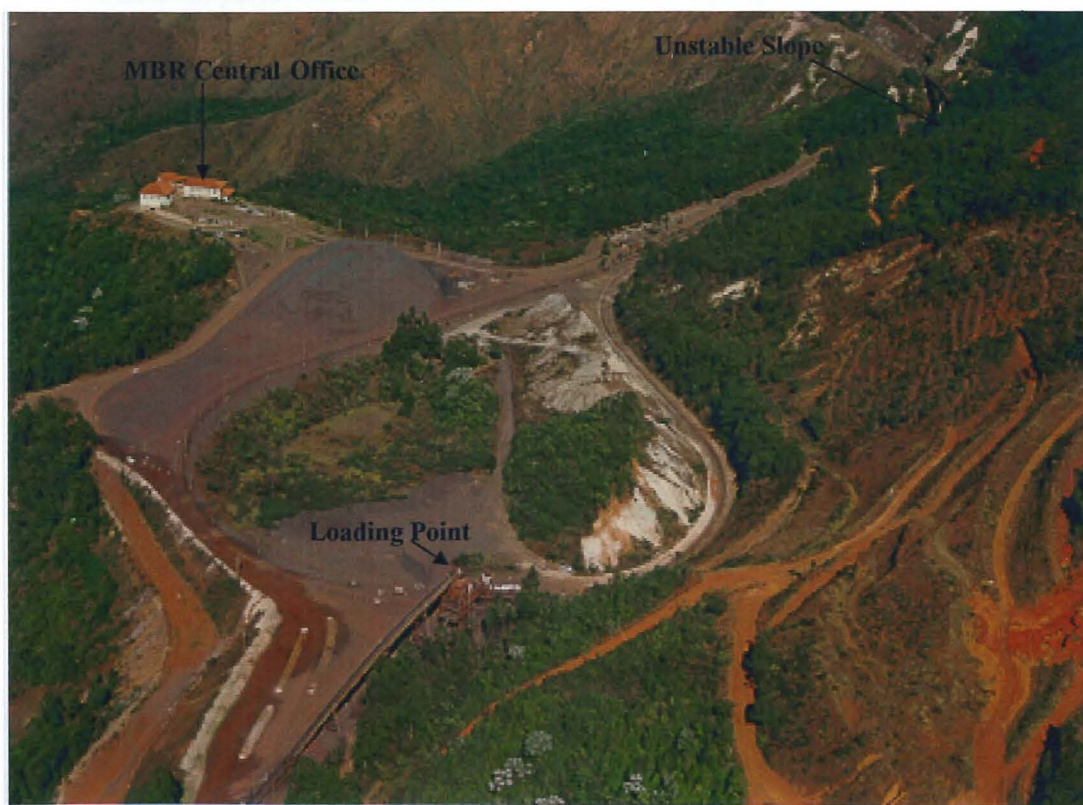
Plate 15 – View of Loading Loop of the Águas Claras Railway Terminal. The development of the railway created instability on the cut slope near the main entrance to the Mine.
