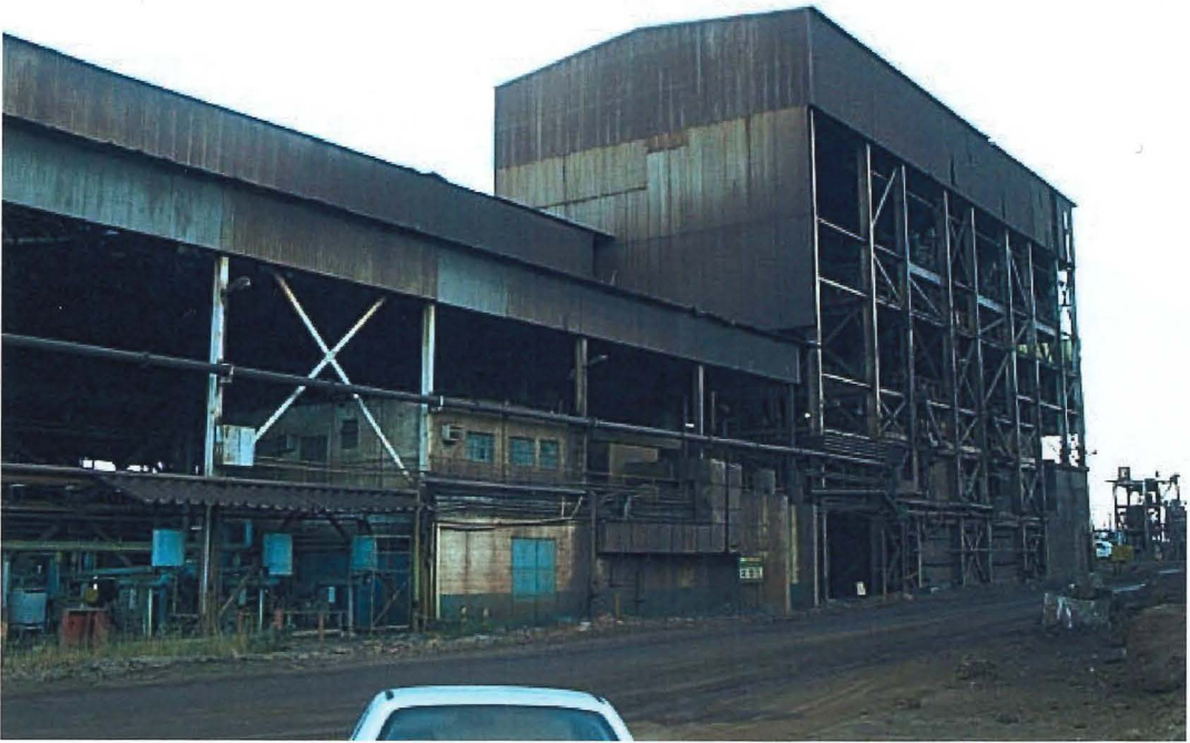
Plate 13 – View of the Águas Claras Ore Processing Plant. (Plate Courtesy MBR).
