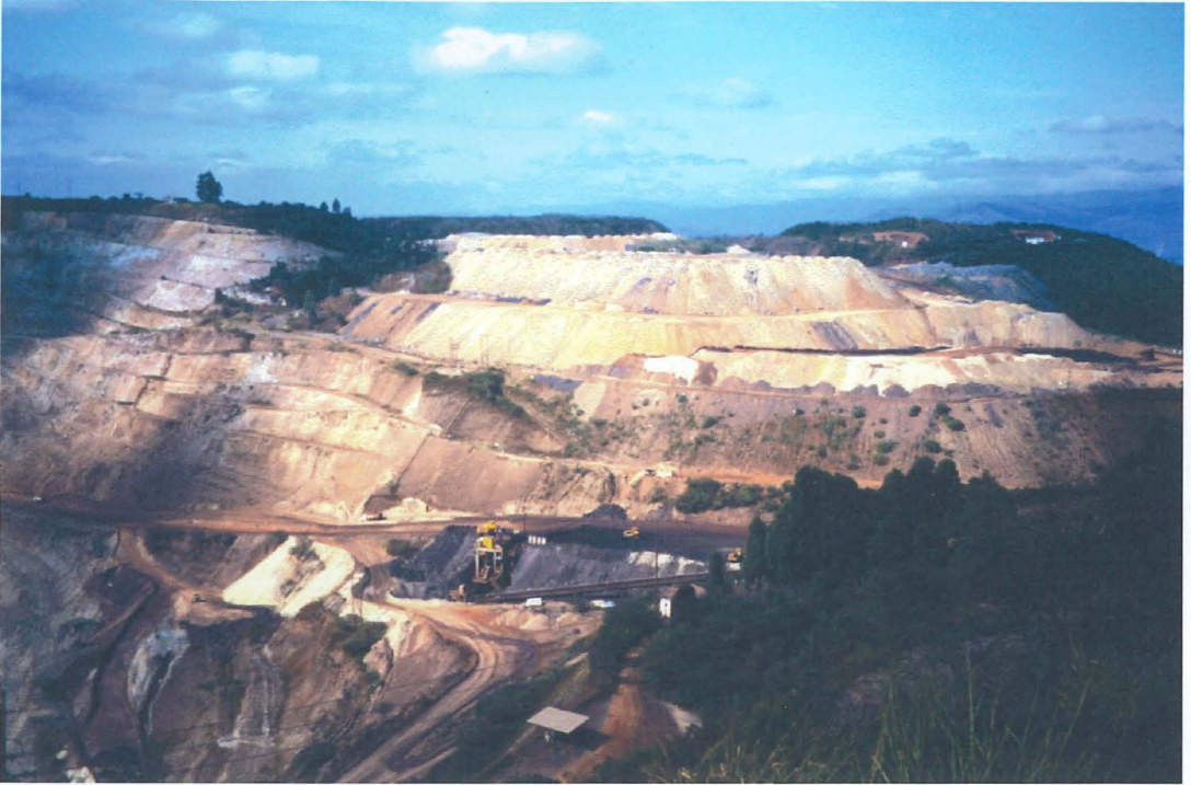
Plate 9 – Top of the Waste Dump, Grota –1, under Construction at the Rim of the Pit.
