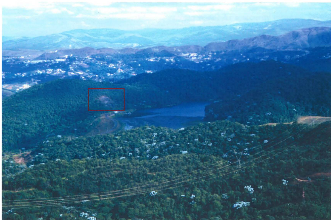
Plate 12 – General View of the Tailings Dam 5. The area inside the red rectangle shows the after effects of the fire that occurred in June 1999.
