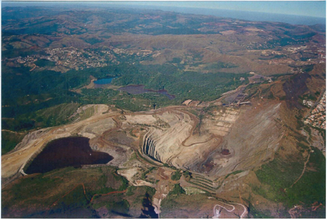
Plate 4 – Aerial View of the PFF Pond. Tailings are pumped from the processing plant to The PFF pond. (Plate courtesy MBR).
