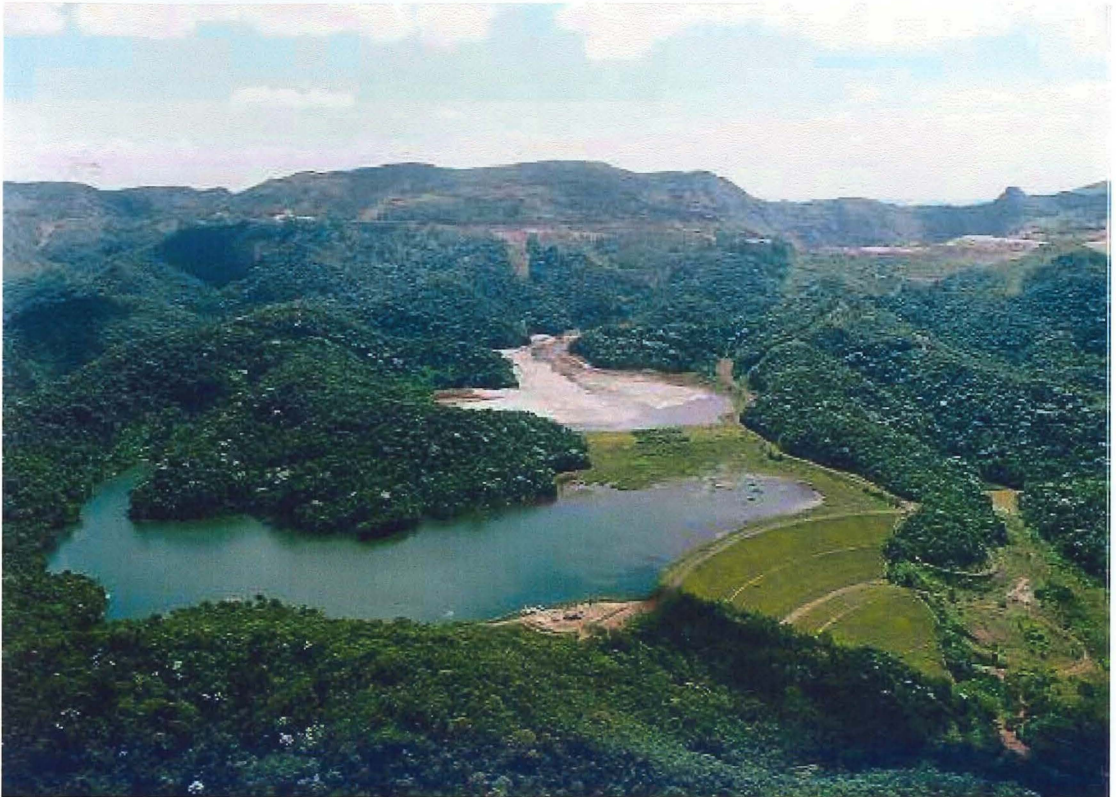
Plate 3 – Aerial View of Águas Claras Tailings Dam 5. Cross-pond dikes are in the centre of the Plate. They divide the pond into two segments, the upper one for tails storage and the lower one specially for reclaiming water. (Plate courtesy MBR).
