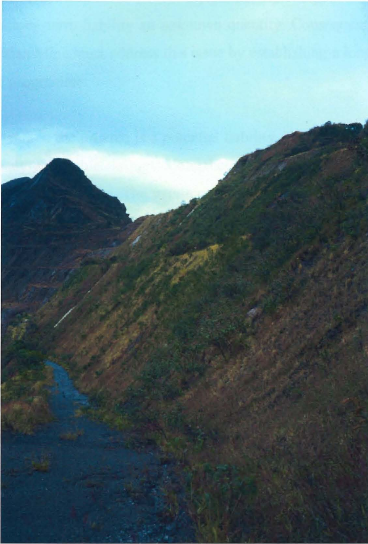
Plate 6 – Steep Slopes Revegetation Process on the North Wall of the Águas Claras Pit.
