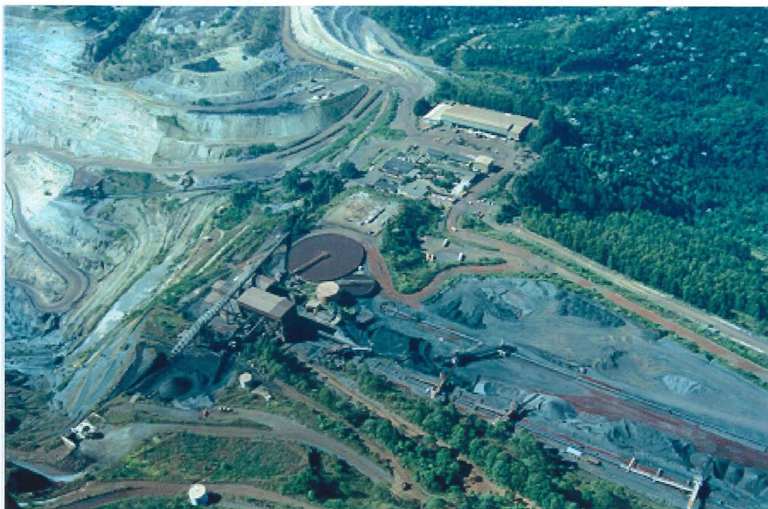
Plate 5 – Aerial View of the Águas Claras Main Facilities. Ore processing plant, heavy equipment garage, restaurant and operational offices can be clearly seen. These facilities will be demolished after the end of the operations and the area rehabilitated. (Plate Courtesy MBR).
