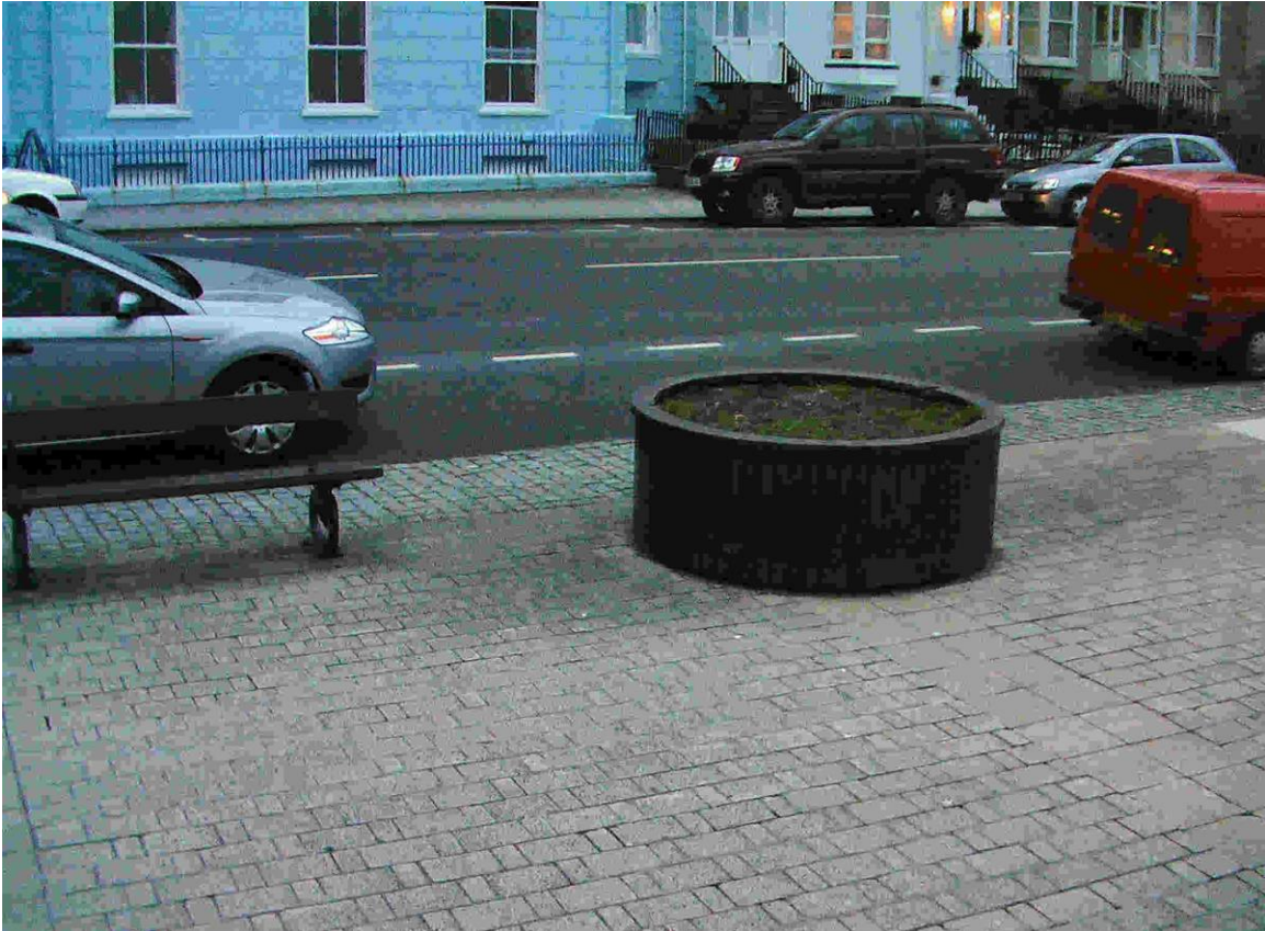
Figure 26: Flowerpot - chain failure – separation.
