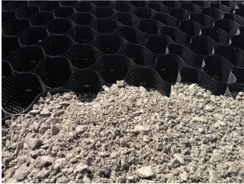
Figure 2.46 Aggregate confinement with geocell and on-site infill. (Presto GeoSystems, 2020)
