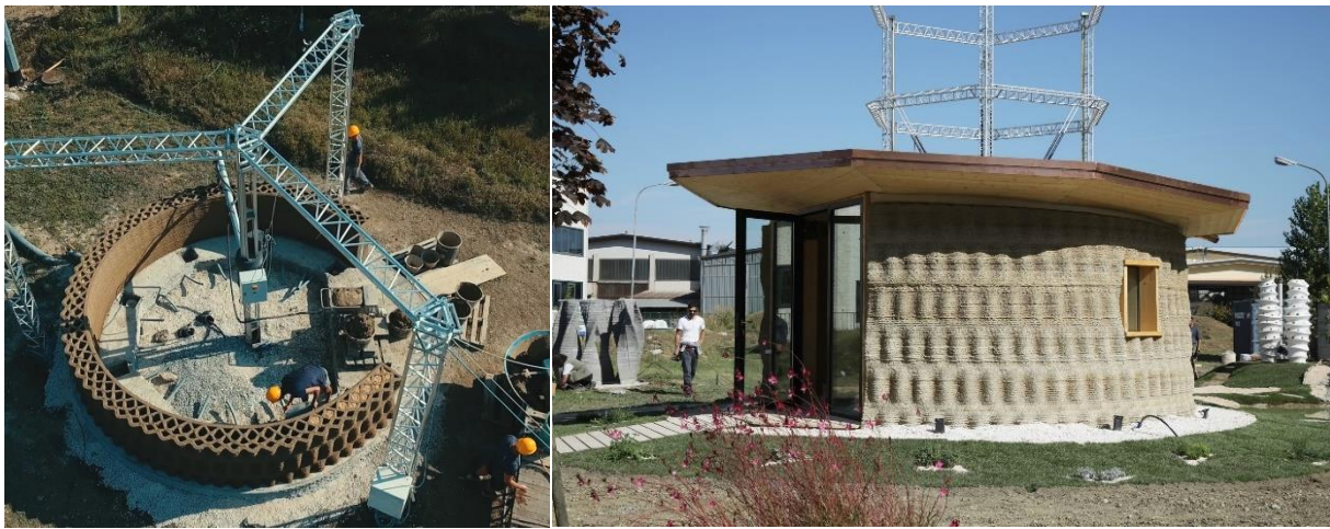
Figure 2.21 The first 3D printed house with earth in Italy (WASP, 2018)
