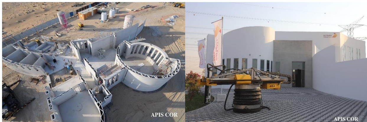
Figure 2.20 The biggest 3D printed building in Dubai (Apis Cor, 2019)
