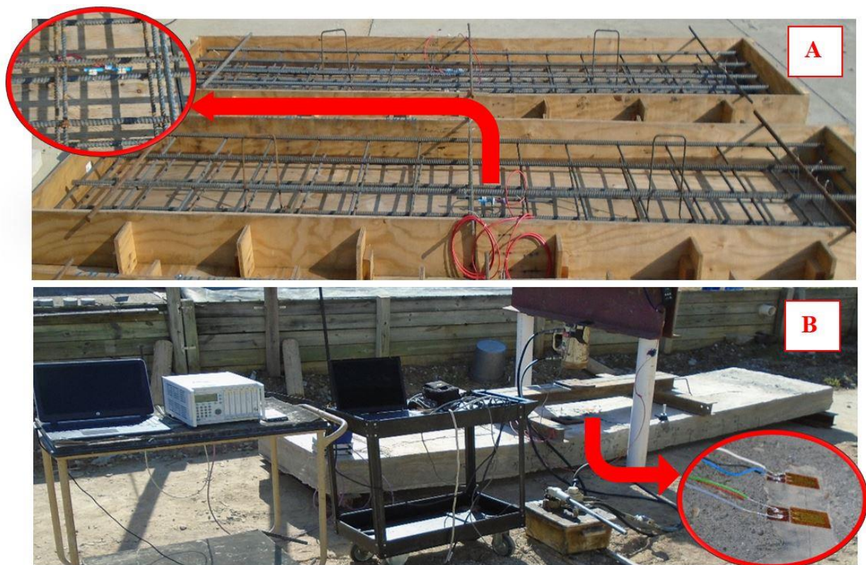
Figure 3-2. Concrete deck fabrication and testing frame.
