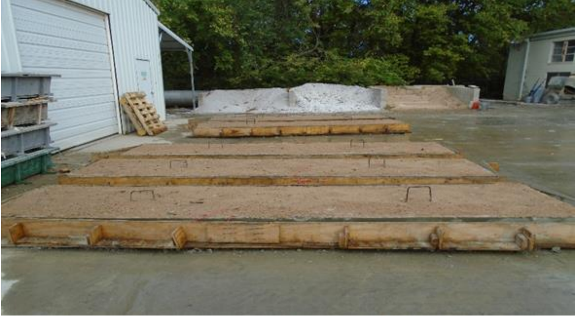
Figure 2-1. Curing of bridge decks.
