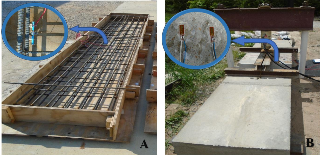
Figure 2-5. Steel and concrete strain gauges.
