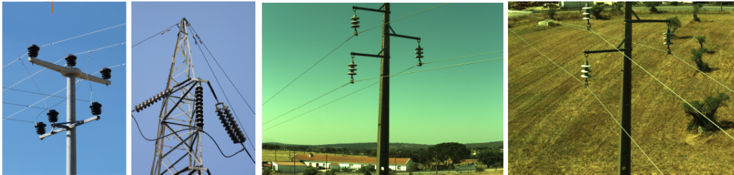
Figure 5.3: Example of images collected by the UAV during the visual inspection.
