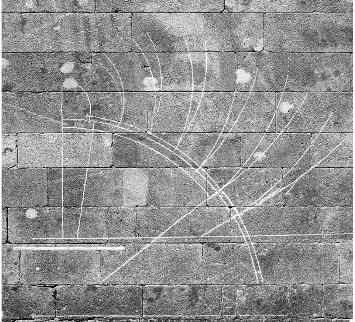
1. Tracings for hemispherical vaults at the parish church of Santa Columba in Carnota. Photograph by Miguel Taín Guzmán
