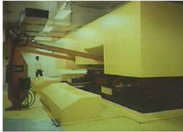
Figura 11 AMS de concreto del edificio Citicorp Center, New York (B. Gallegos 2014)
