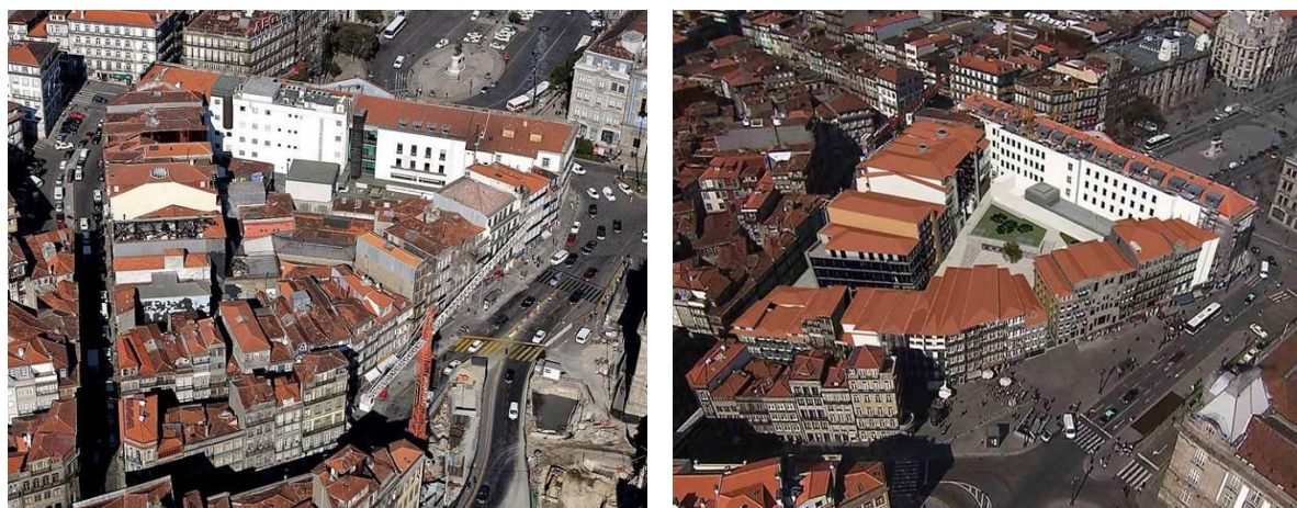
Figure 4 – « Cardosas » neighbourhood before ( https://jpn.up.pt/wp-content/uploads/2015/03/20090921-cardosas3.jpg ) and after intervention ( http://www.fa-arquitectos.pt/portfolio/quarteirao-das-cardosas/ ).
