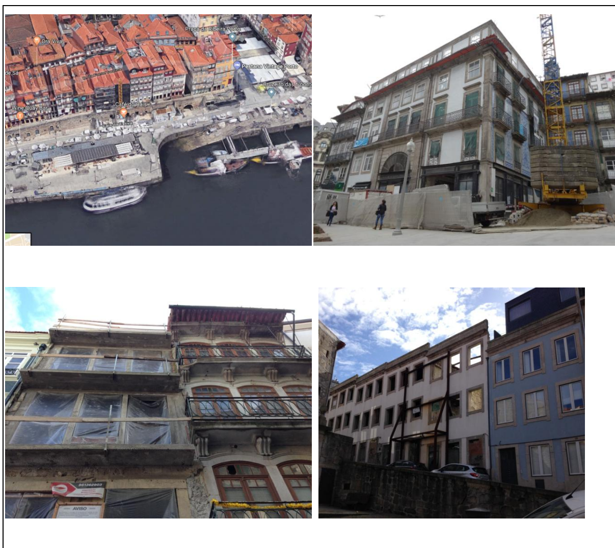
Fig. 13. Other completed and ongoing works :
