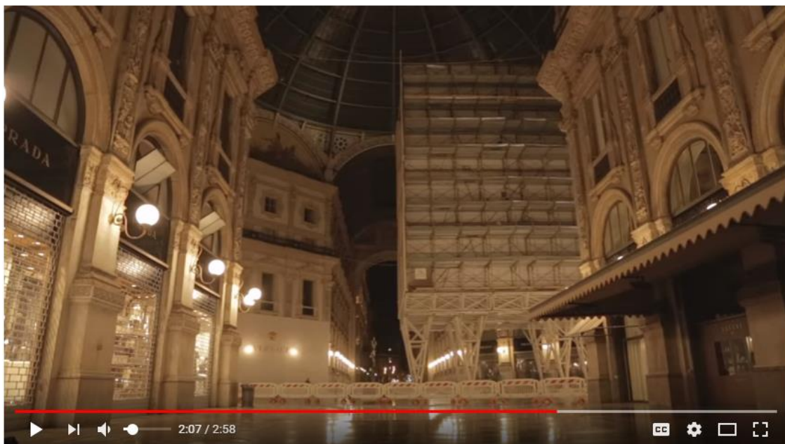
INGALLERIA - Completing the restoration project
