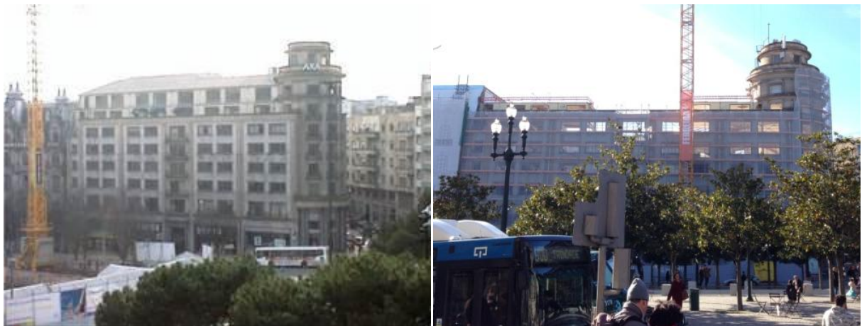
Figure 9 – Building Seguros Garantia, at Aliados Avenue, before ( http://mipweb.cm-porto.pt/MuniSIG/dados/cva/jpgs/Si12.jpg ) and during intervention (Soraya Genin, 2018)
