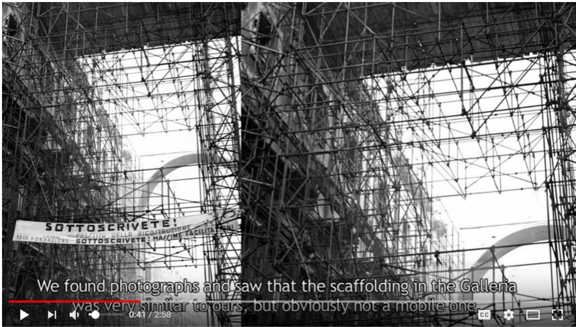
INGALLERIA - Completing the restoration project
