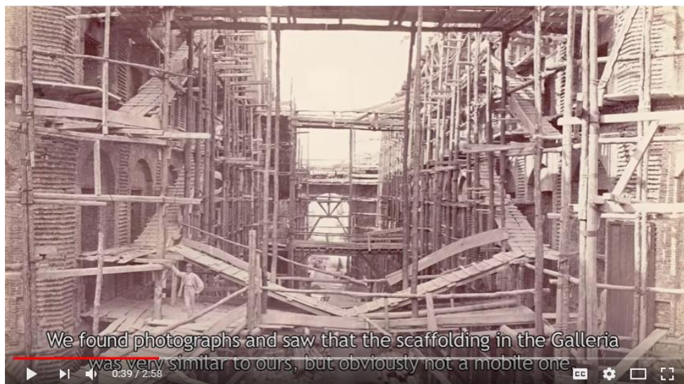
INGALLERIA - Completing the restoration project
