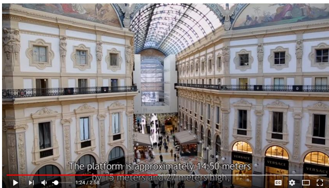
INGALLERIA - Completina the restoration project
