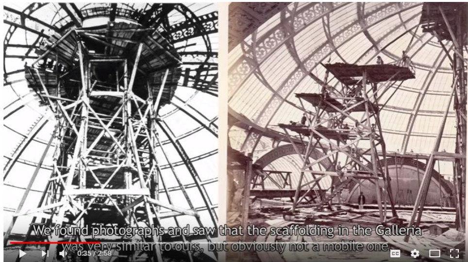
INGALLERIA - Completing the restoration project
