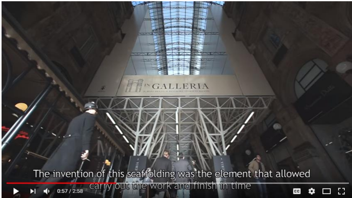
INGALLERIA - Completing the restoration project
