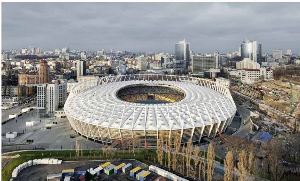
Figure 4. 11.: Olimpiyskiy National Sports Complex, Ukraine. An example of a tension-structured roof (Schlaich Bergermann Partner, 2011).
