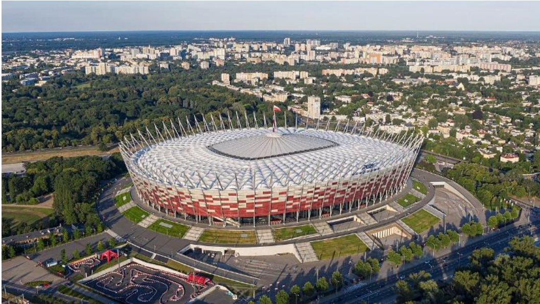
Figure 4. 12.: Stadion Narodowy w Warszawie, Poland. An example of an air-supported roof (Wikipedia, 2019).
