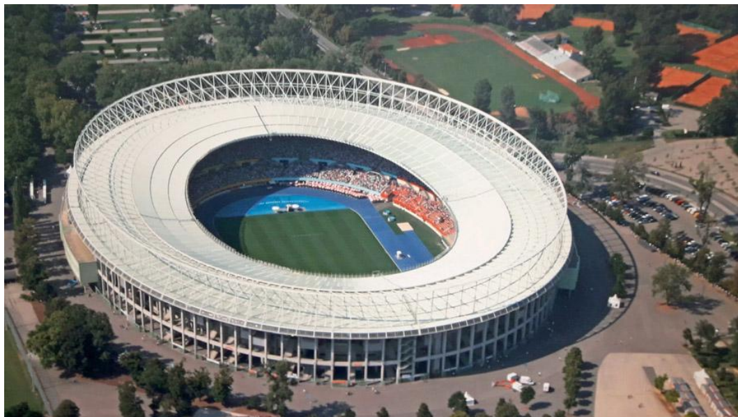
Figure 4. 10.: Ernst-Happel-Stadion , Austria. An example of a compression/tension ring (Sport-Österreich, 2017).
