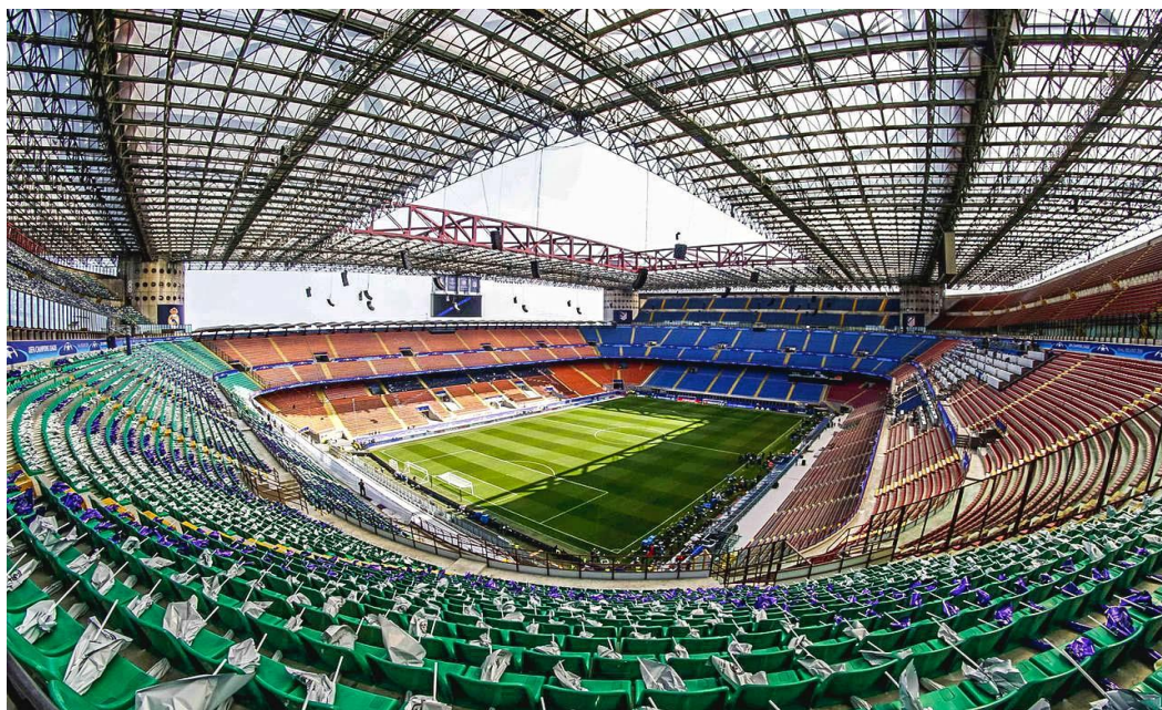
Figure 4. 13.: Stadio Giuseppe Meazza, Italy. An example of space frames (Rappo, 2019)
