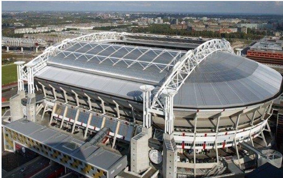
Figure 4. 14.: Johan Cruijff Arena, Netherlands. An example of a retractable roof (Holland Online, 2018)
