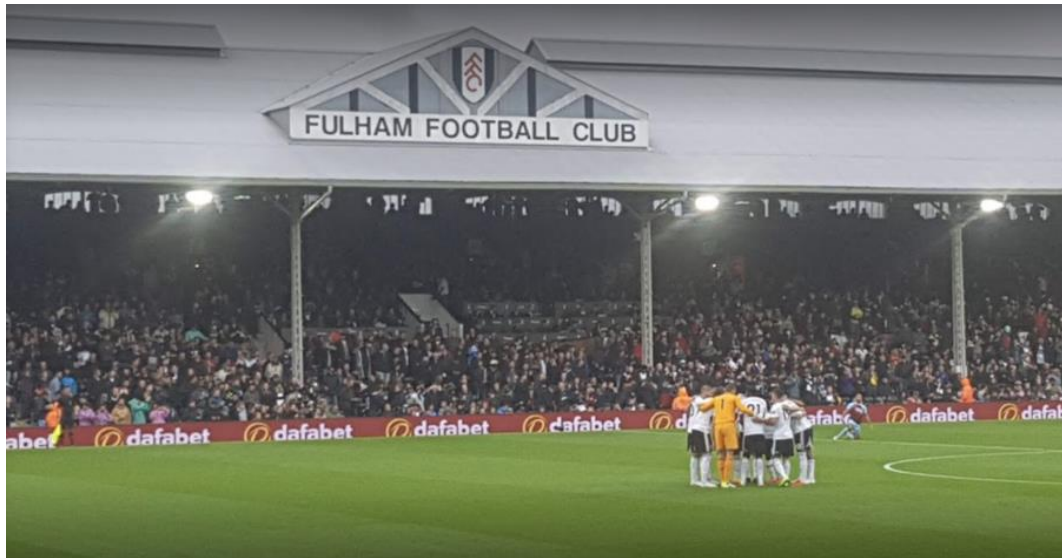
Figure 4. 6.: Craven Cottage, England. An example of post and beam structures (Stadium Journey, 2019).
