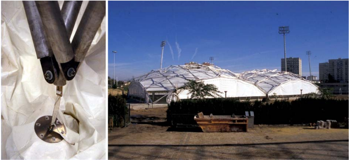
Figure 2.- San Pablo swimming pool: a linkage and the deployed roof.
