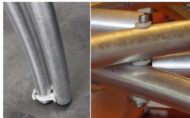
Figure 22: Detail of joint with Teflon washers
