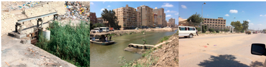
Figure 3. The Mahmoudia Canal in Egypt. Source: Author. Legend: The downstream end of the canal, located nearby a police station, is surrounded by garbage heaps ( left ); the bank earth of the canal is mixed with garbage, located in front of the water plant of Alexandria ( middle ); the water plant viewed from the canal ( right ). Location: 31^{\circ}11'05.6'' N 29^{\circ}52'55.4'' E ( left ), 31^{\circ}13'14.6'' N 29^{\circ}59'27.4'' E ( middle and right ).
