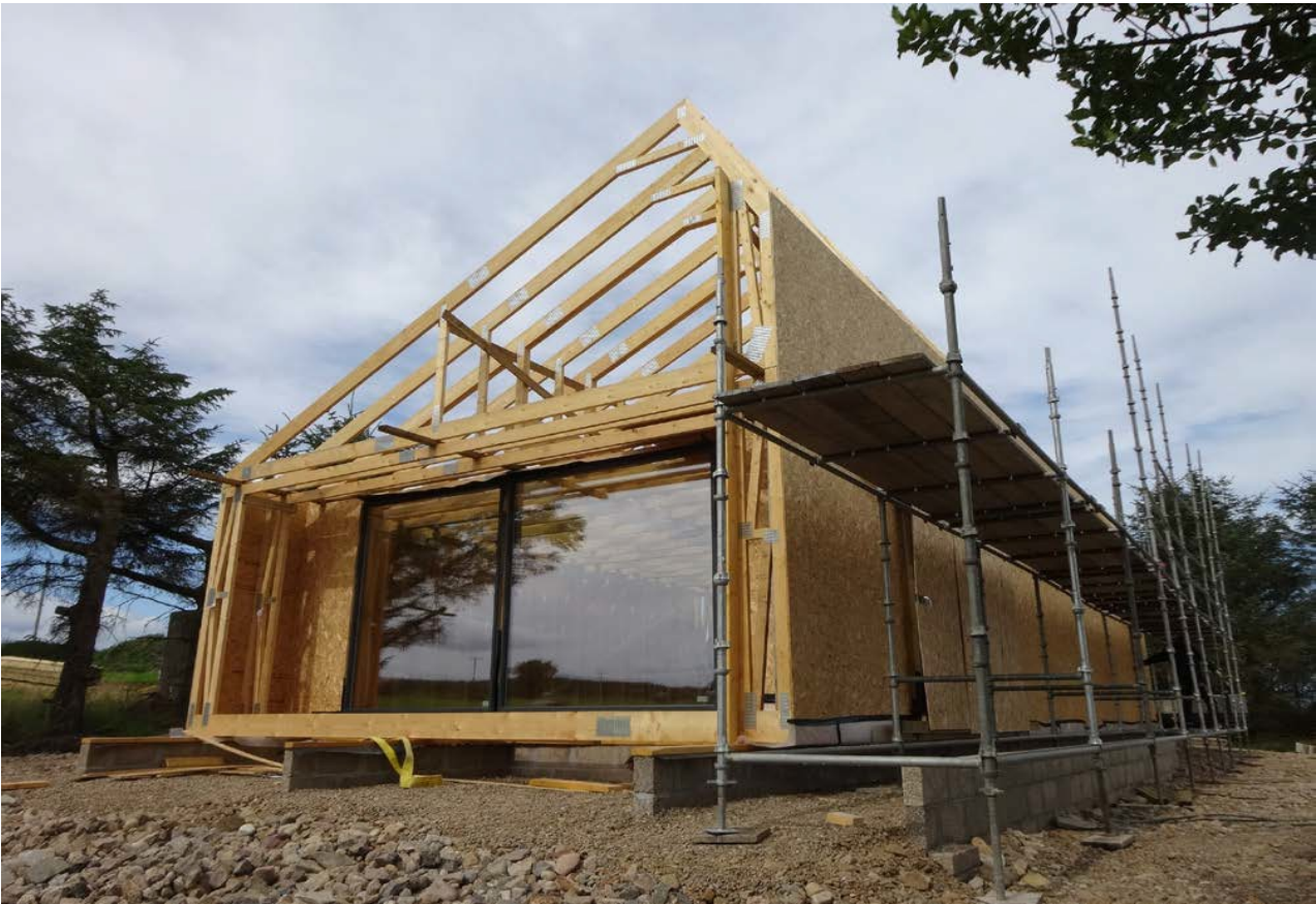
Fig. 6. Ground floor and first floor trusses put in place
