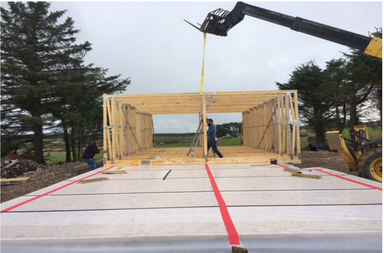
Fig. 5. Two men are enough to assemble the whole house
