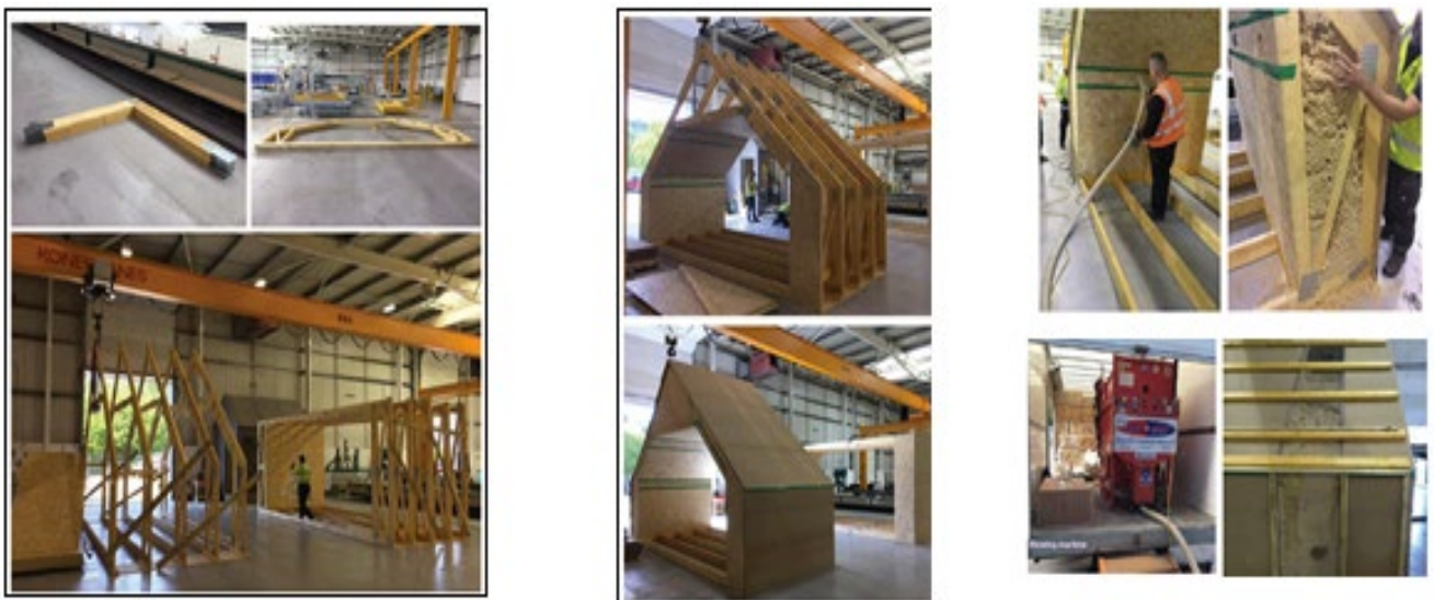
Fig. 3. Workshop tests of trusses & wood blown insulation at Hamilton, CSIC.
