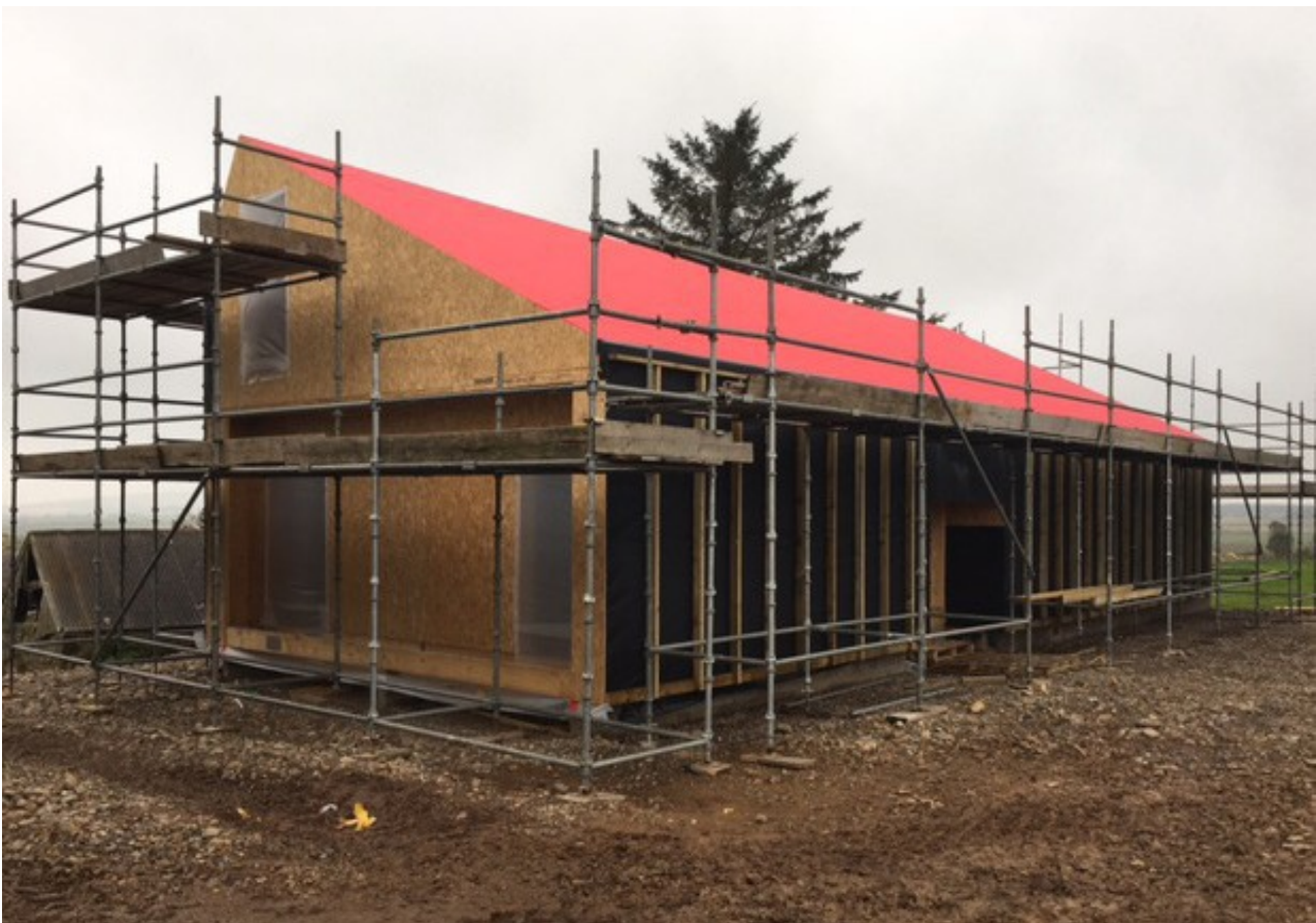
Fig. 7. The water-tight Integra House typology
