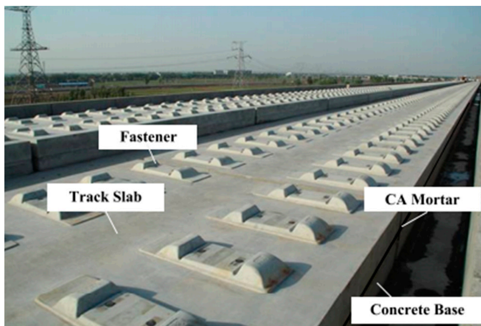
Figure 4. Cement Asphalt (CA) mortar under a slab track (with permission from American Society of Civil Engineers (ASCE)) [33].
