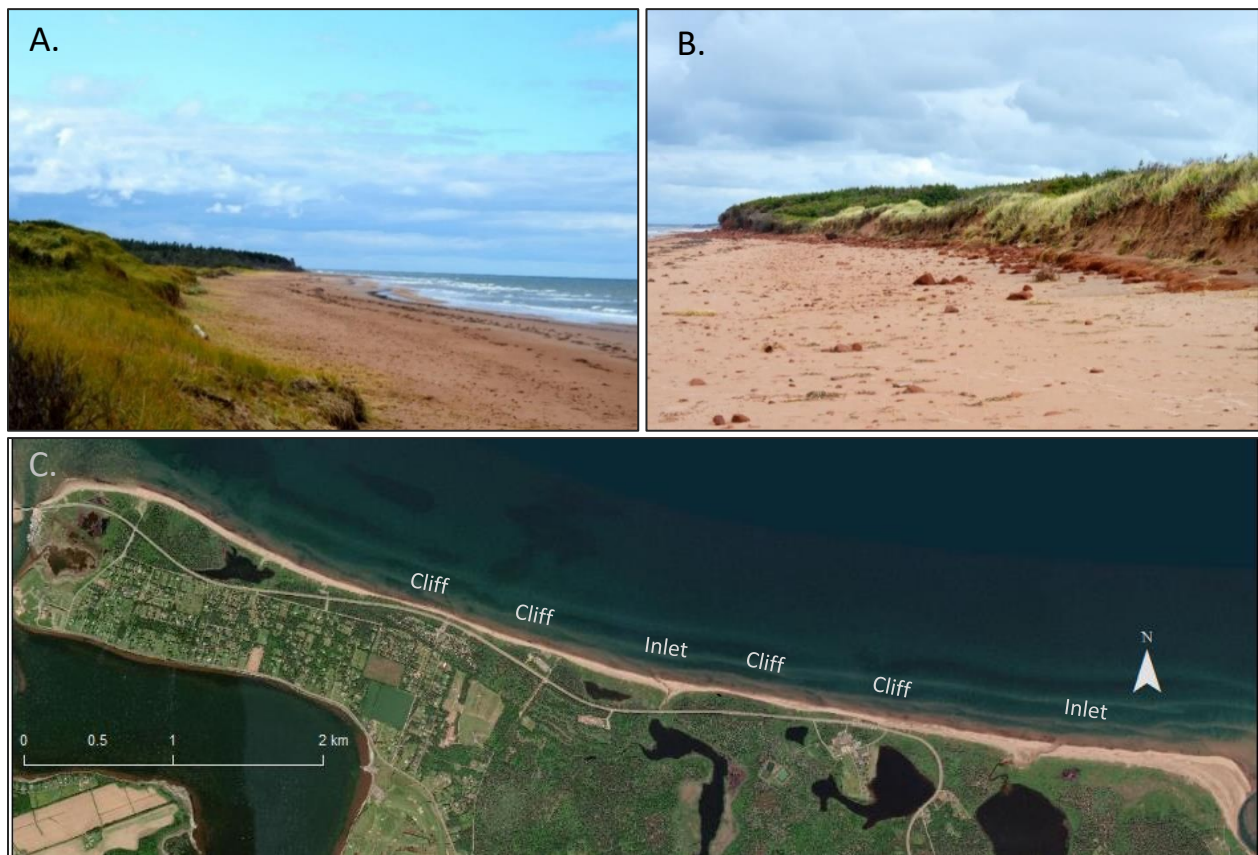
Figure 7. A. September 2019 image showing the low continuous foredunes of Stanhope beach. B. September 2019 image of a bluff alongshore of Stanhope beach. C. ArcGIS map of Stanhope beach.
