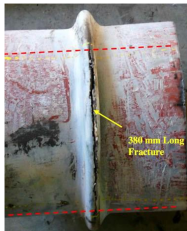
Figure 1.2: Fractured Field Pipeline of Husky Energy Inc. (Courtesy of Husky Energy Inc.)
