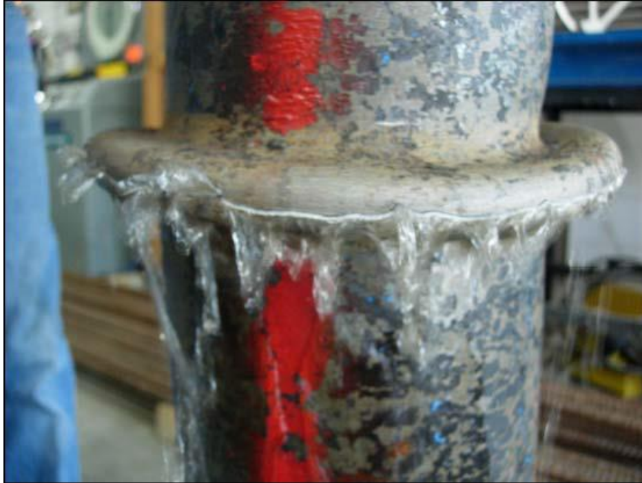
Figure 2.9: Rupture Failure of Wrinkled Pipe (Nazemi et al., 2009)
