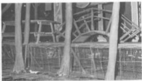
Bridge, picnic table in place. Wire mesh ready for foam.
