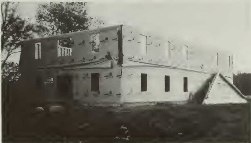
Exterior framing for first & second floor
