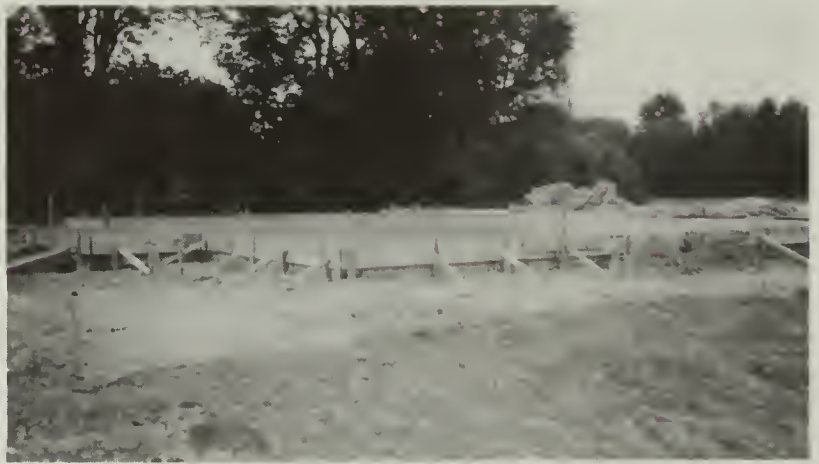
Concrete slab work
