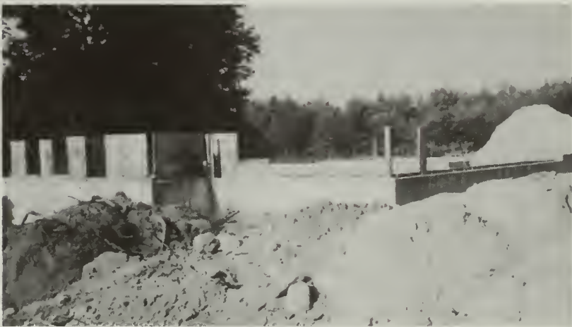
Foundation for New Town Hall
