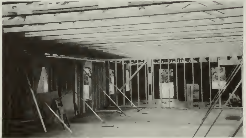
Interior framing of first floor
