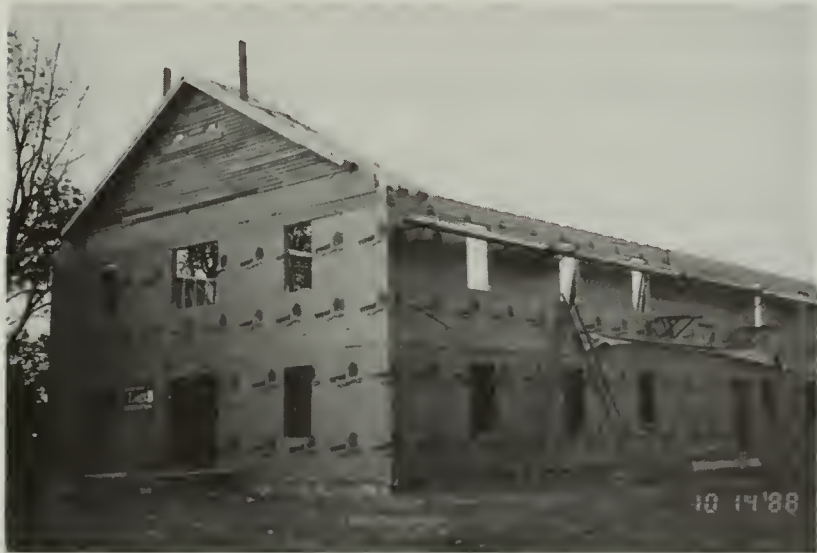
Gable end in place
