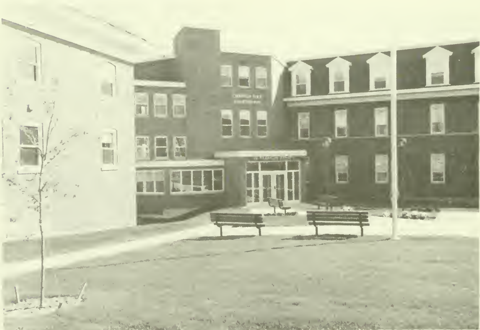
A new look at the corner of Franklin and Green Streets — the former St. Martin Church/School/Convent/Rectorry Site now converted to the 49-unit elderly housing complex — CHARPENTIER APARTMENTS , a $2.6 million development undertaking by the Somersworth Housing Authority.
