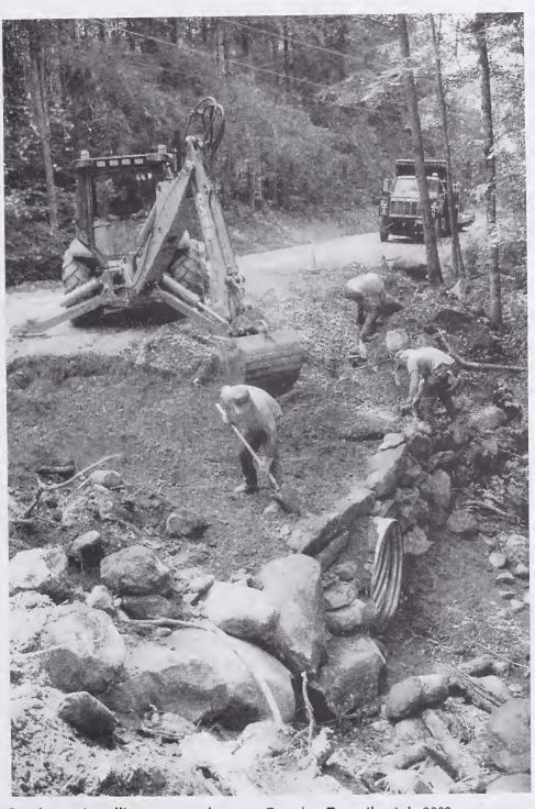
Road crew installing a new culvert on Croydon Turnpike, July 2003.
