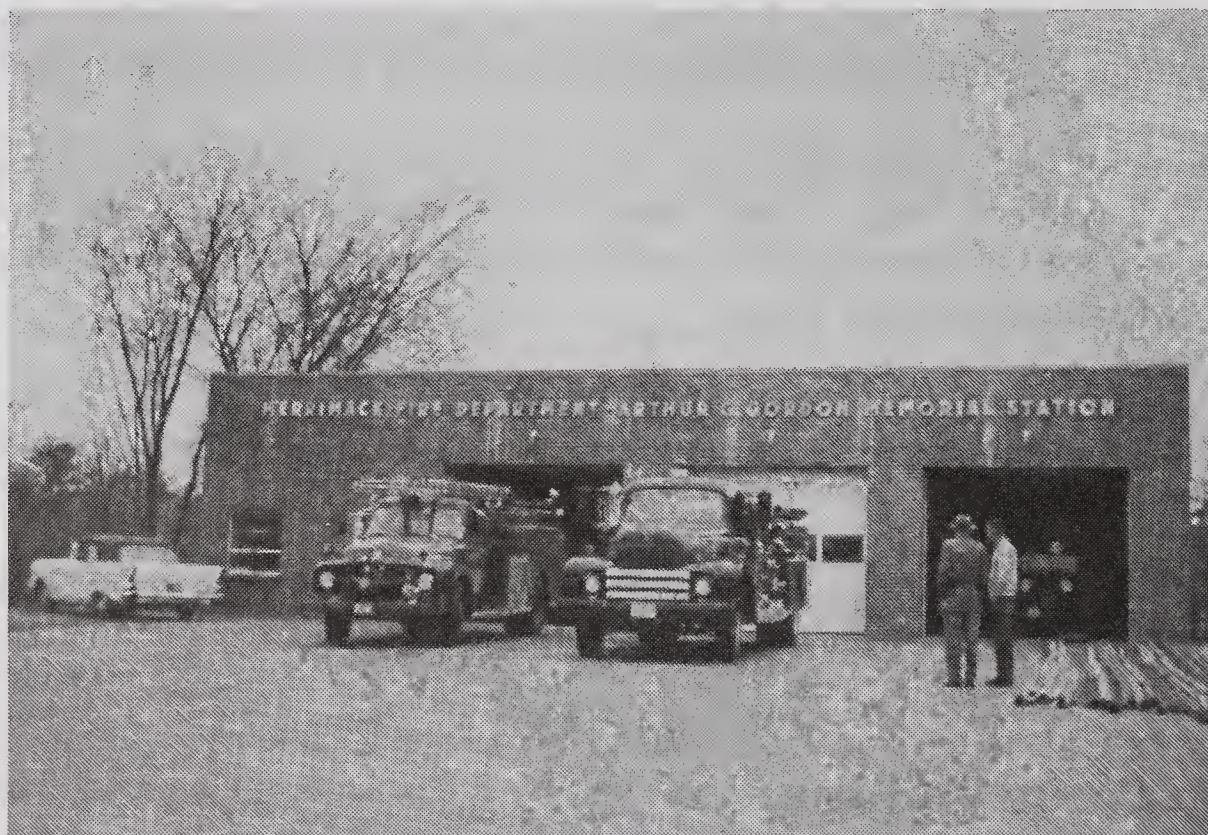
Central Fire Station on Route 3 before the addition was added.
