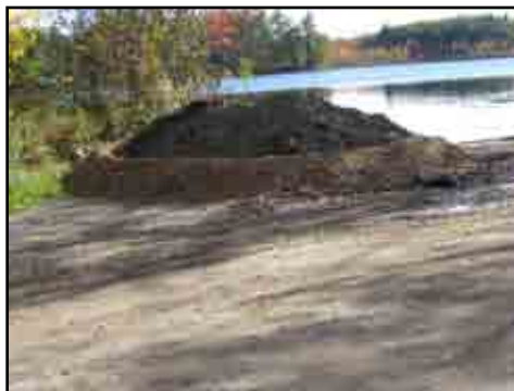
FLINTS POND EROSION CONTROL AT NH FISH AND GAME BOAT LAUNCH
