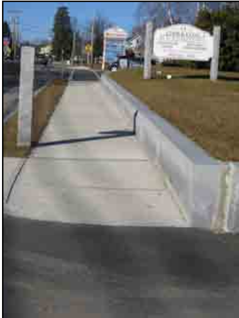
A SECTION OF THE ASH STREET SIDEWALK
