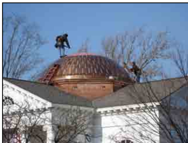
PUTTING THE FINISHING TOUCHES ON THE LIBRARY ROOF
