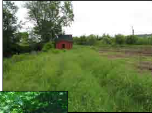
CLEARING BEGINS ON WOODMONT WEST PHOTO: HEATHER JUSSEAUME
