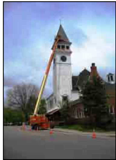
ROOFING THE CLOCK TOWER PHOTO: CATHY HOFFMAN
