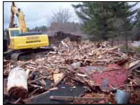
BUILDING DEMOLITION AT WOODMONT
