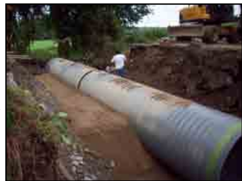
DOW ROAD CULVERT REPLACEMENT
