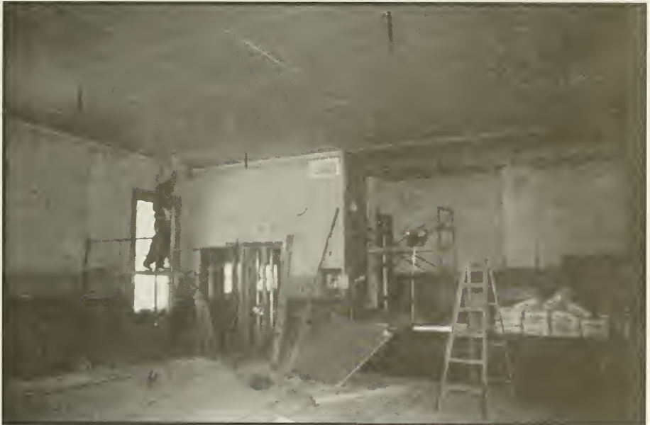
Ceiling restoration at the Grasmere Town Hall.
