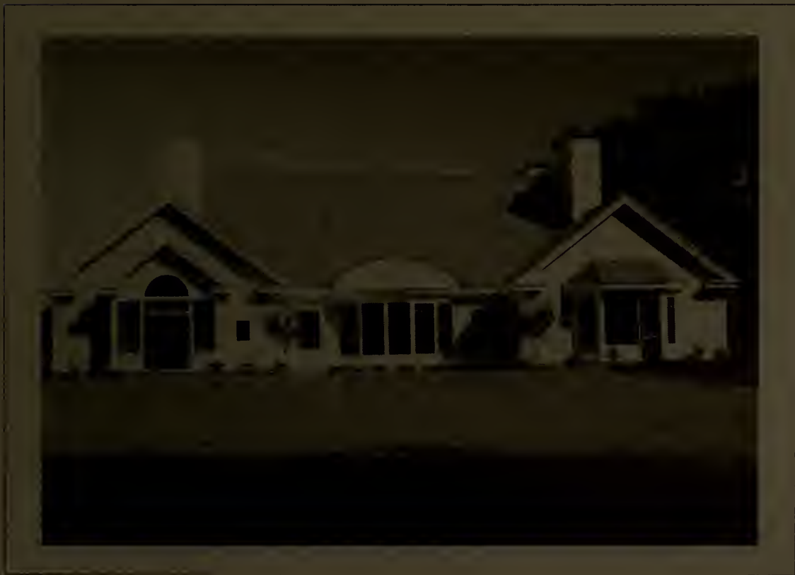
New Fremont Public Library - Built 2002
