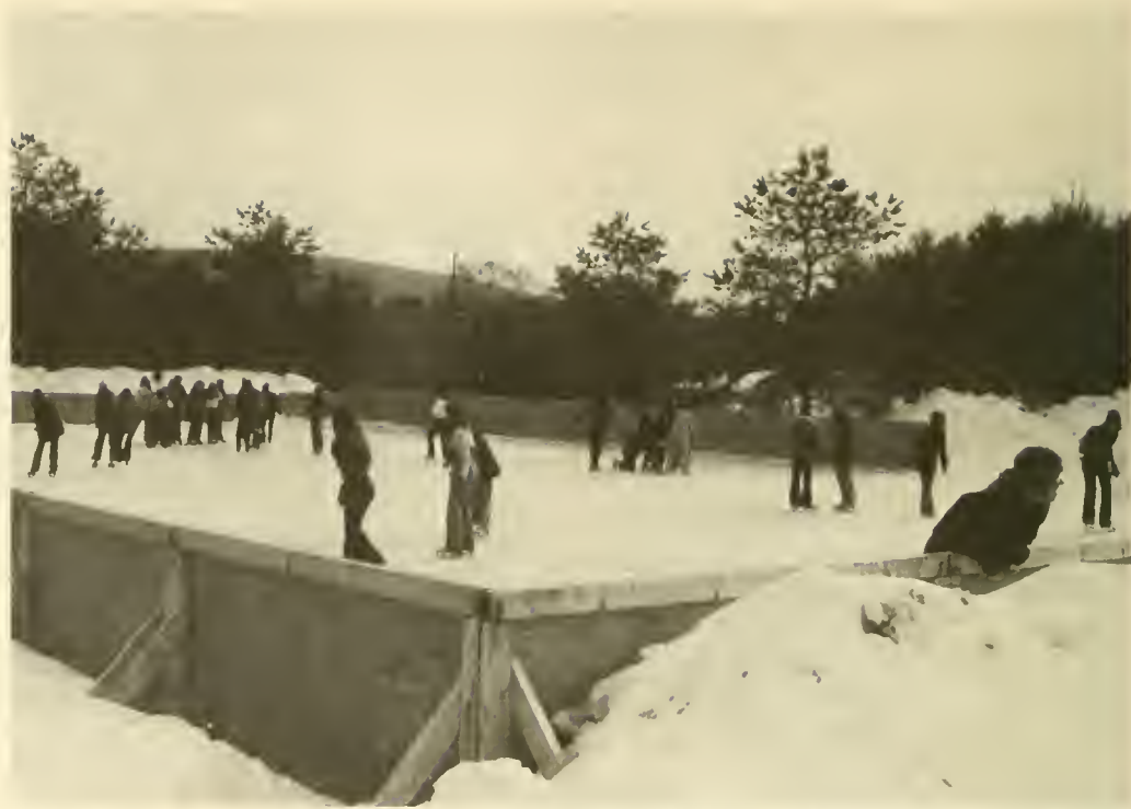
Newly Constructed Skating Rink at Recreation Center Parks & Playgrounds.
