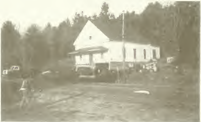
Renovation on Town Hall
