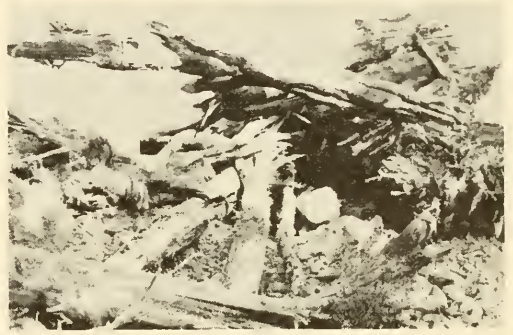
DEBRIS REMOVED FROM UNACCEPTABLE ROAD BED
