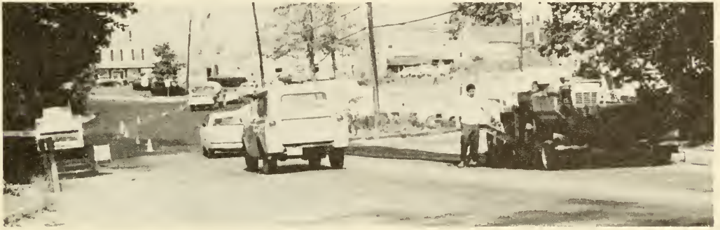
MILL ROAD PAVING
