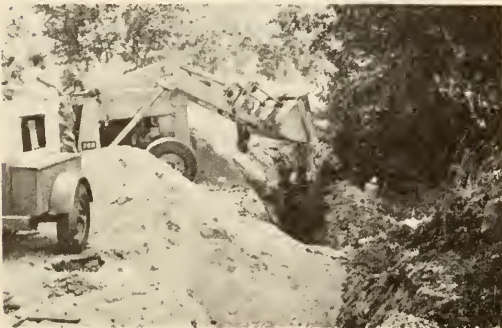
TOWN CREW INSTALLING WATER PIPE ON EMERSON ROAD
