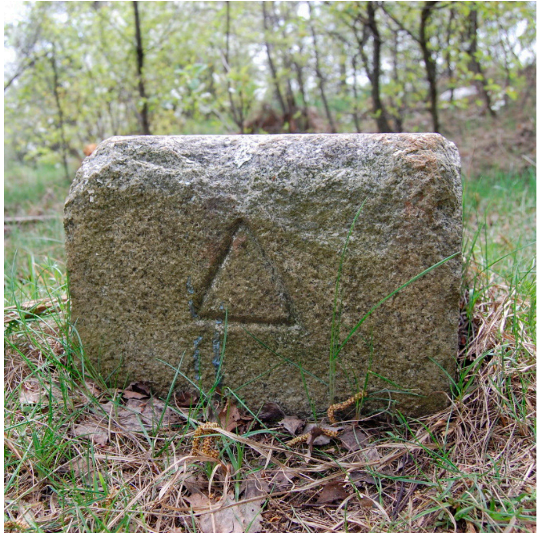
Figure 3. The astrogeodetic mark “Sucha Góra”.
